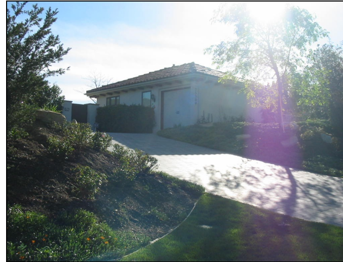
View of the second entrance and secondary housing unit.
