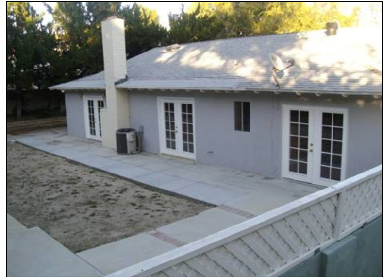
Picture after the addition had been removed and restored the home back to its original condition.
