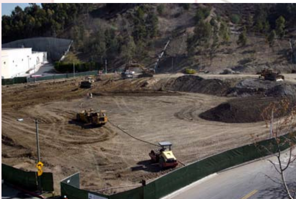
Site during grading
