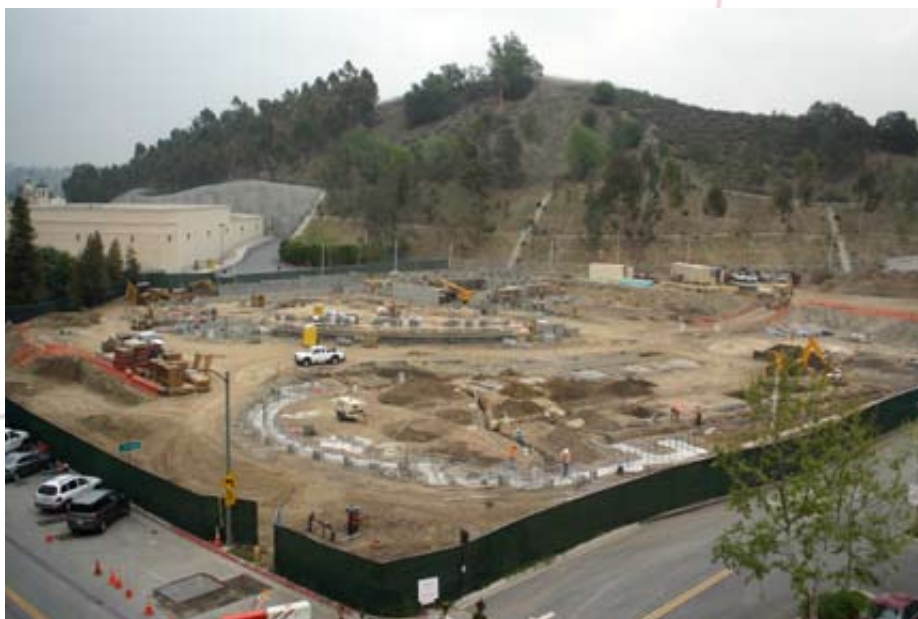
Site during foundation work
