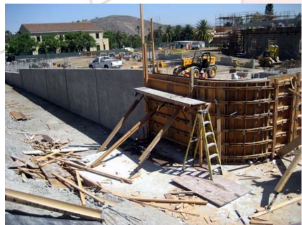
forms for poured in place site wall
