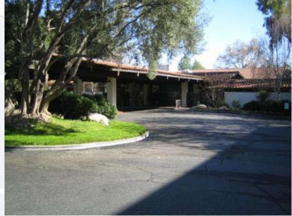
Existing Calabasas Inn building
