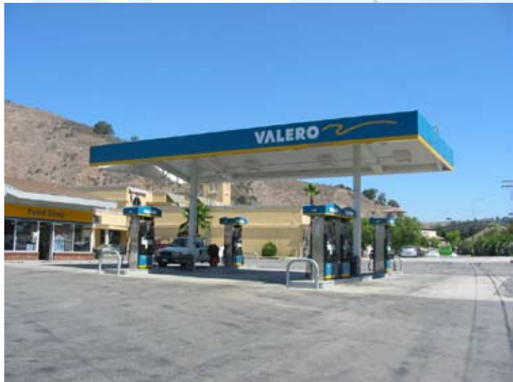
Top & Above: Views of the existing service station
