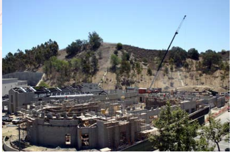
Site during steel construction
