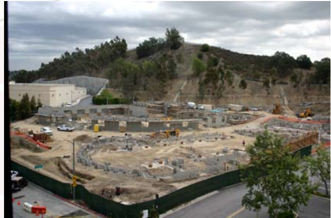
Site at beginning of wall construction
