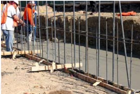
Crew checks reinforcing bar in foundation
