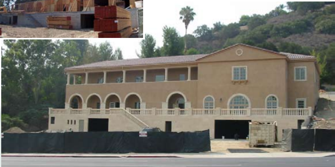
Views during the framing (top) and near completion of the project
