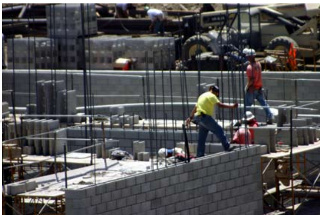
Crew checks wall reinforcing bars
