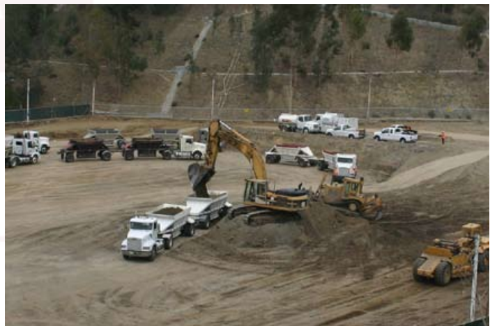
Grading included removing expansive soils from the site
