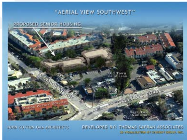
Aerial view showing project
