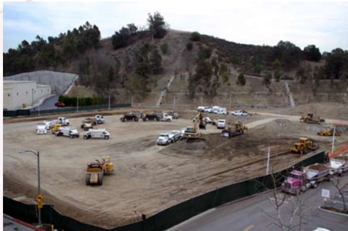
Site during grading
