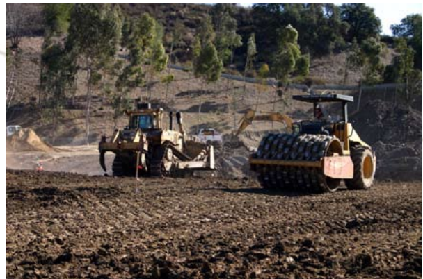
Grading occurring on the site
