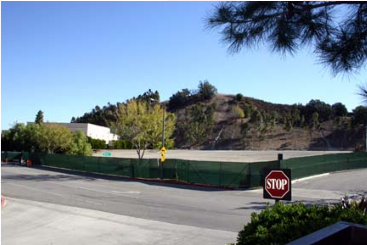
Site prior to grading
