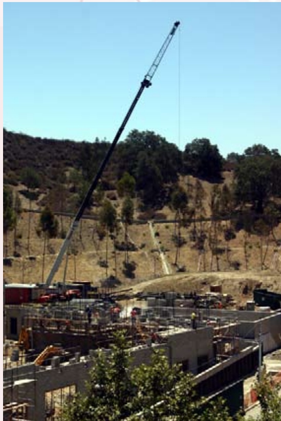
Crane lifting concrete block into location
