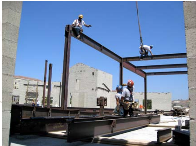
Crew secures beam in place
