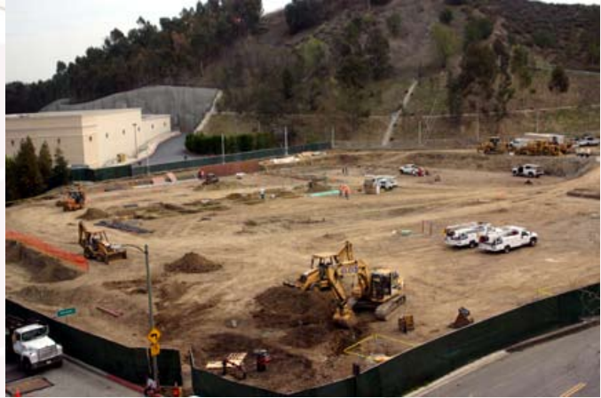
Site at beginning of foundation work
