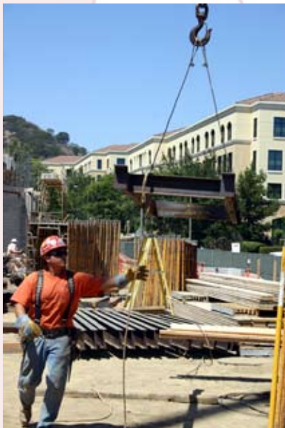
Crew lifts beam into location
