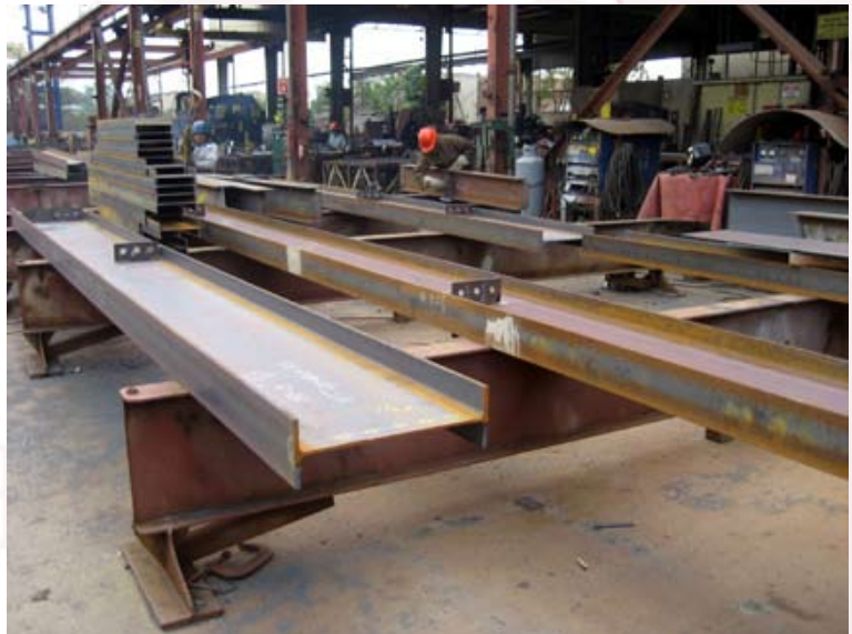
Steel for Civic Center at factory
