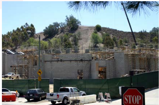
Walls of the new City Council Chambers
