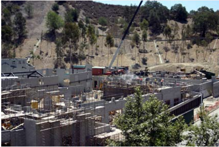
Construction of City Hall Walls
