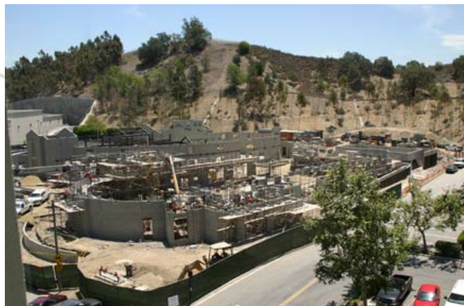
Site during wall construction
