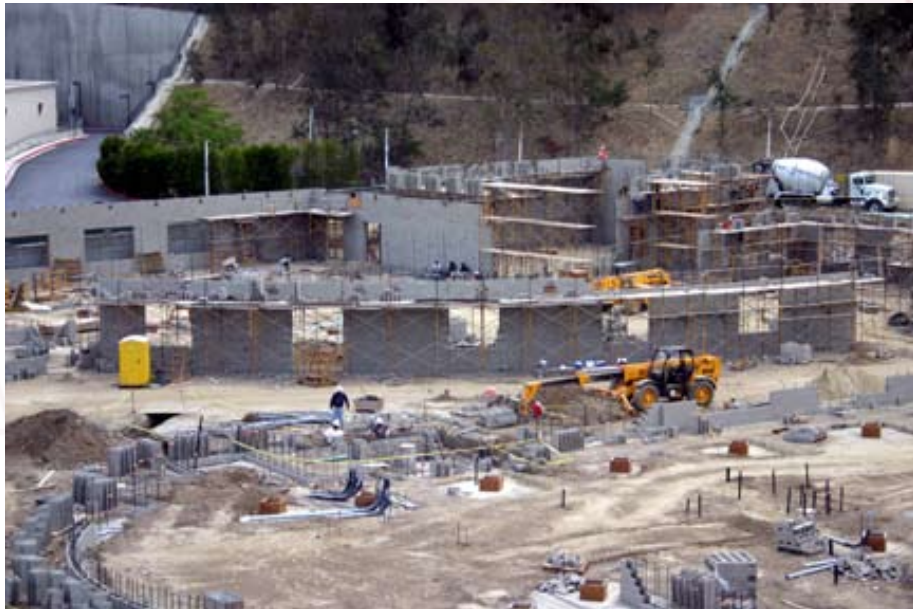
Crew begins construction of City Hall walls (library in background)
