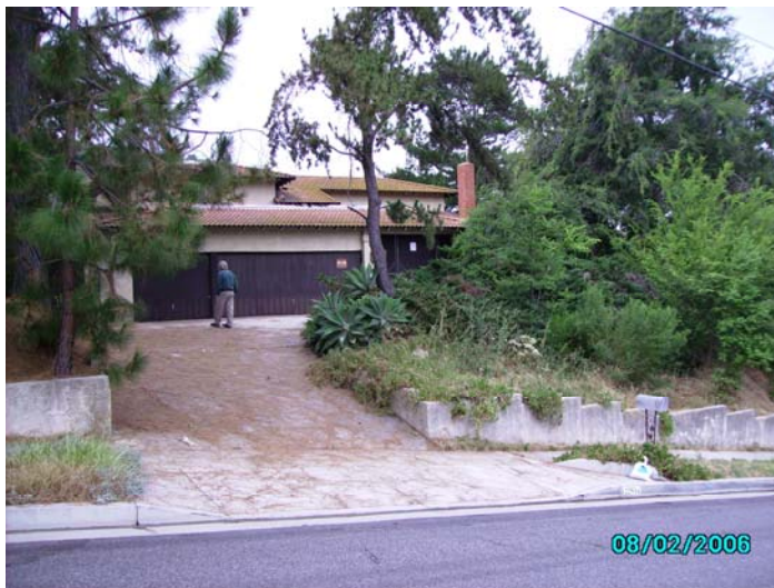
Overgrown/ Dilapidated property causing a Public Nuisance.
