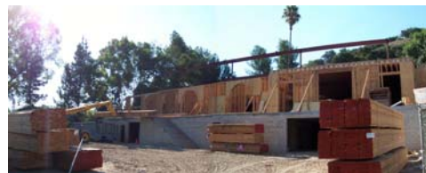
First City Funding Building under construction
