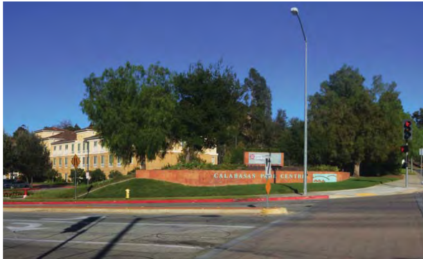
Photo 1: Looking east at the project site from across Park Sorrento.
