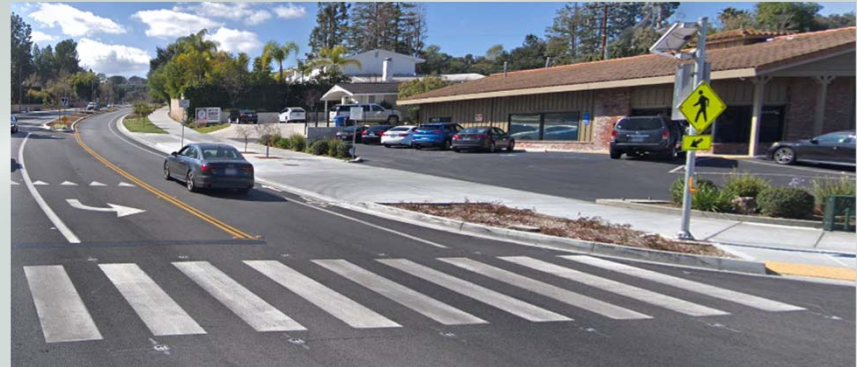
In-Road Pavement Lights
