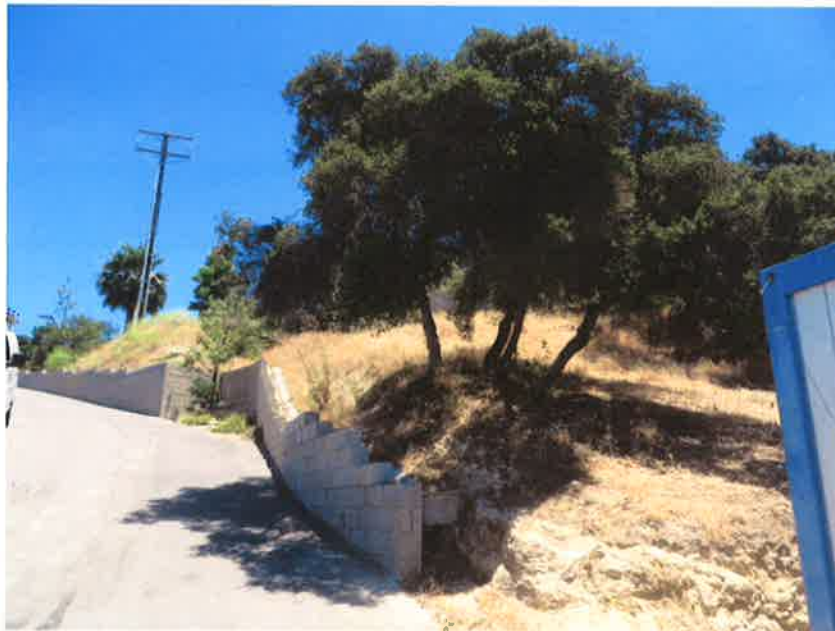
Scrub Oak #20 is located near the east property boundary above the site, Fern Trail Dr., and previous retaining wall. It is encroached by a new retaining wall and drain line within the west protection zone/dripline. Grade cuts should be done by hand and monitored. Looking east.
