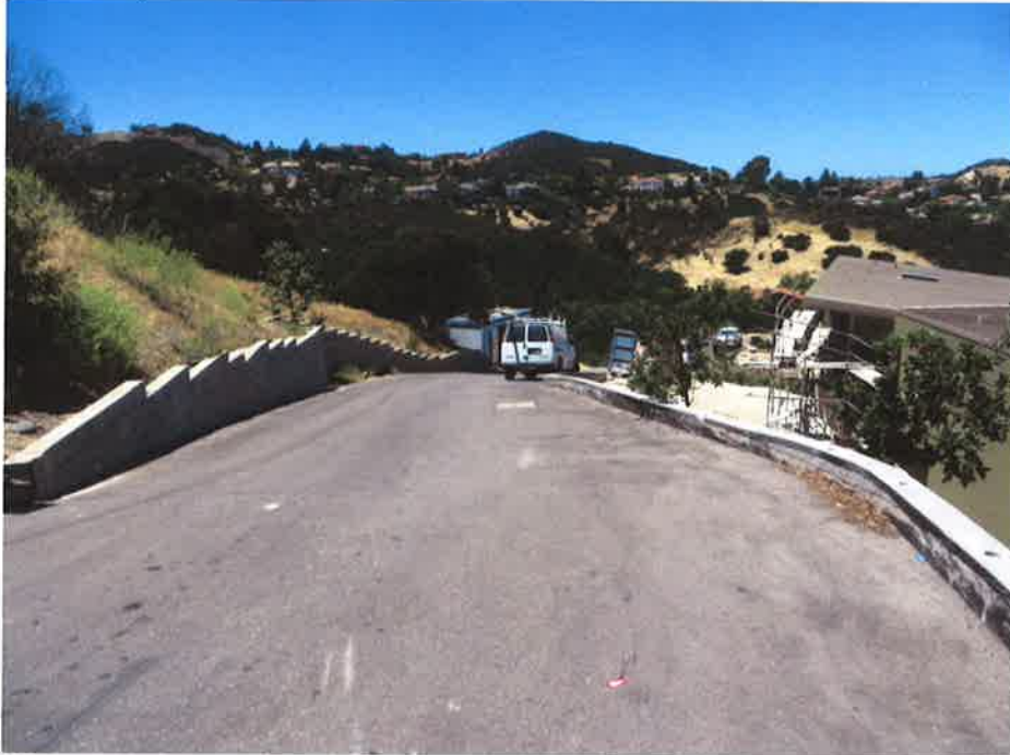
Looking west down fern Trail to the site left of the parked van. Three new homes are at right.
