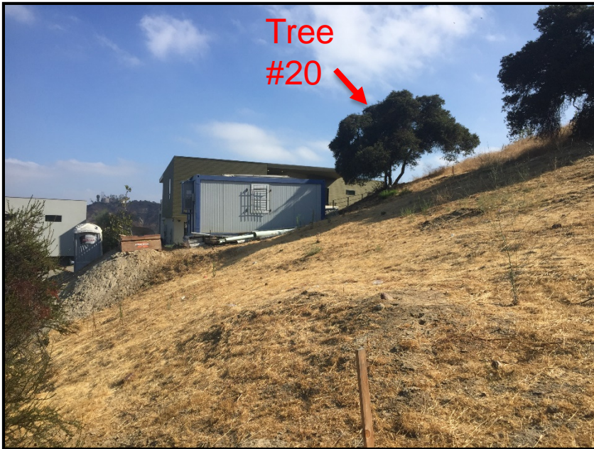
1. Overview of 23472 Fern Tr. property lot, standing in SW corner, view facing NE corner of property. Scrub oak Tree No. 20 is at northeast property boundary and will be encroached upon by a new retaining wall during construction.
