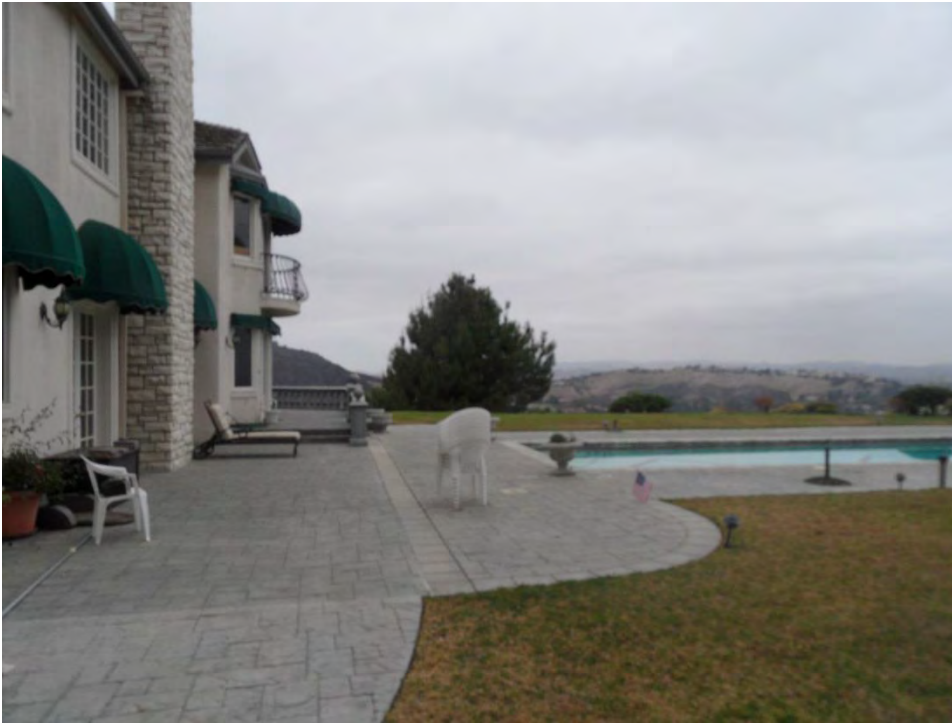
Rear elevation, facing west
