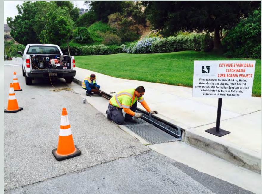
Completion of Citywide Catch Basin Curb Screen Project
