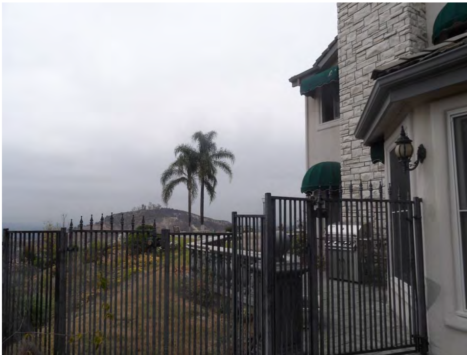
Side elevation, facing north
