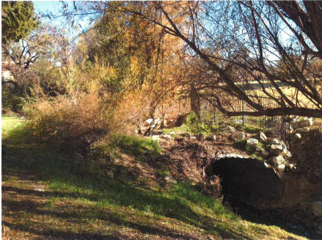
Northeast view – existing dirt path over CMP culvert
