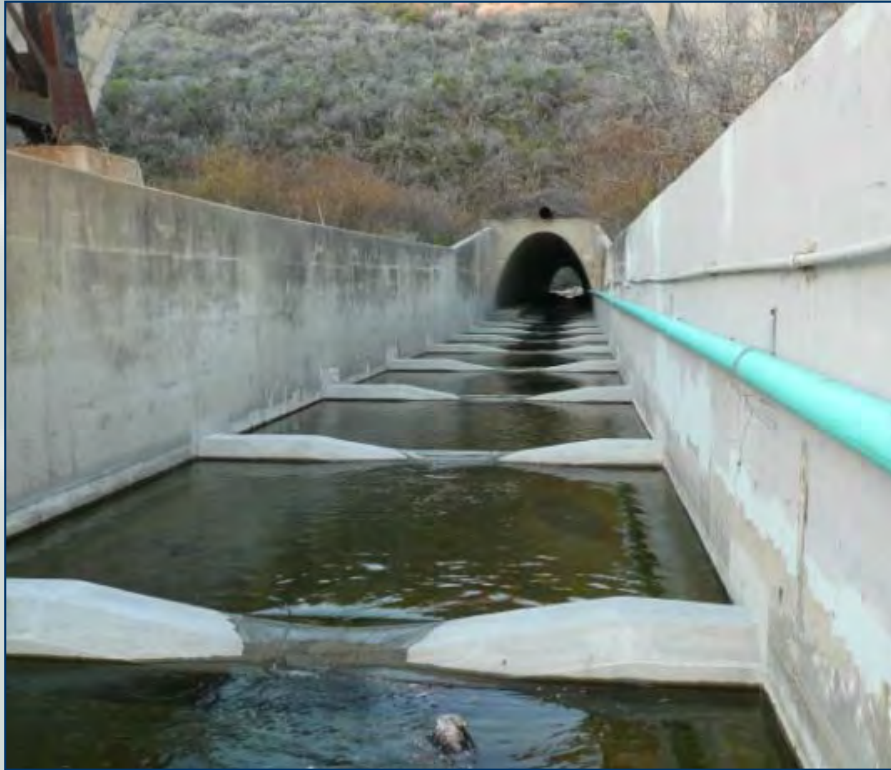
Baffles in structure
