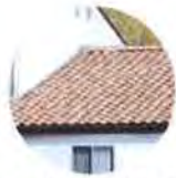
• "S" Tile Roof
