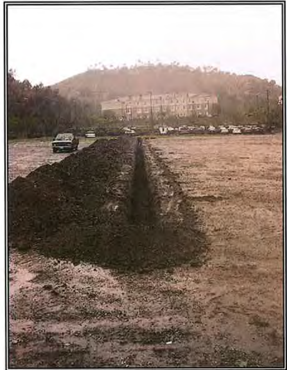
Photo 1: Test Trench T-15, View west
