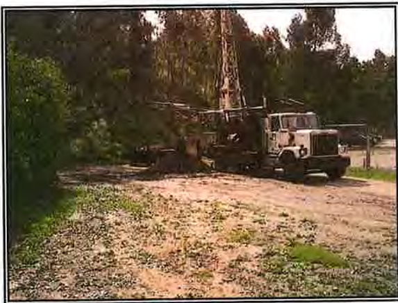
Photo 2: Boring B-8 near southeast portion of site taken on 3-20-05.
