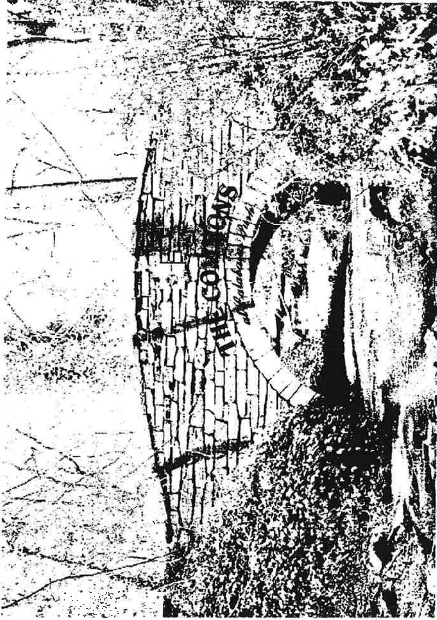
1/2" THICK FLAT CUT OUT LETTERS EITHER NATURAL BRONZE OR BRONZE PETINA FINISH - PIN SET OF FACE OF BRIDGE (FINAL COLOR TO BE DETERMINED)
