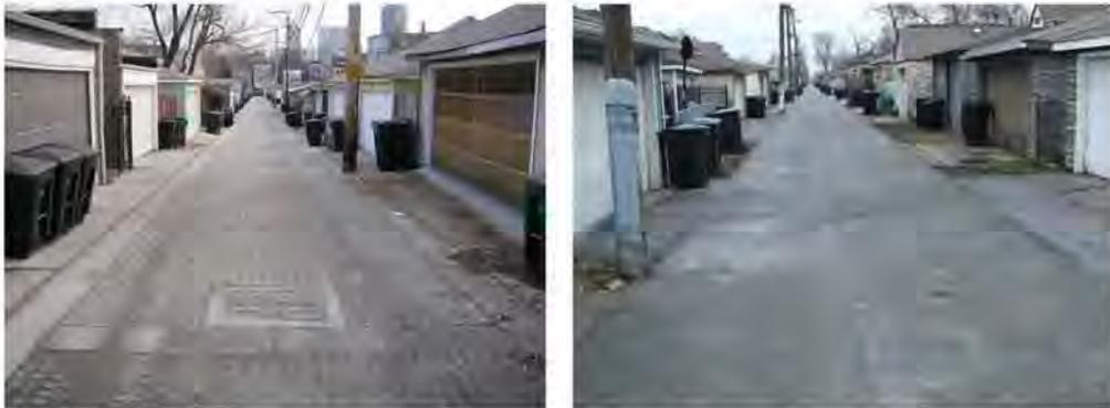
**Figure 10: Permeable Pavers and Permeable Concrete Chicago Alleys**
