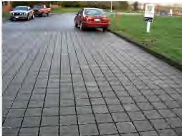
Figure 3. Permeable pavers used in the roadway of a neighborhood development in Wilsonville, OR
