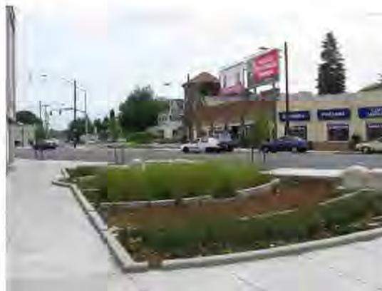
**Figure 2. This bioretention area takes runoff from the street through a trench drain in the sidewalk as well as runoff from the sidewalk through curb cuts**
