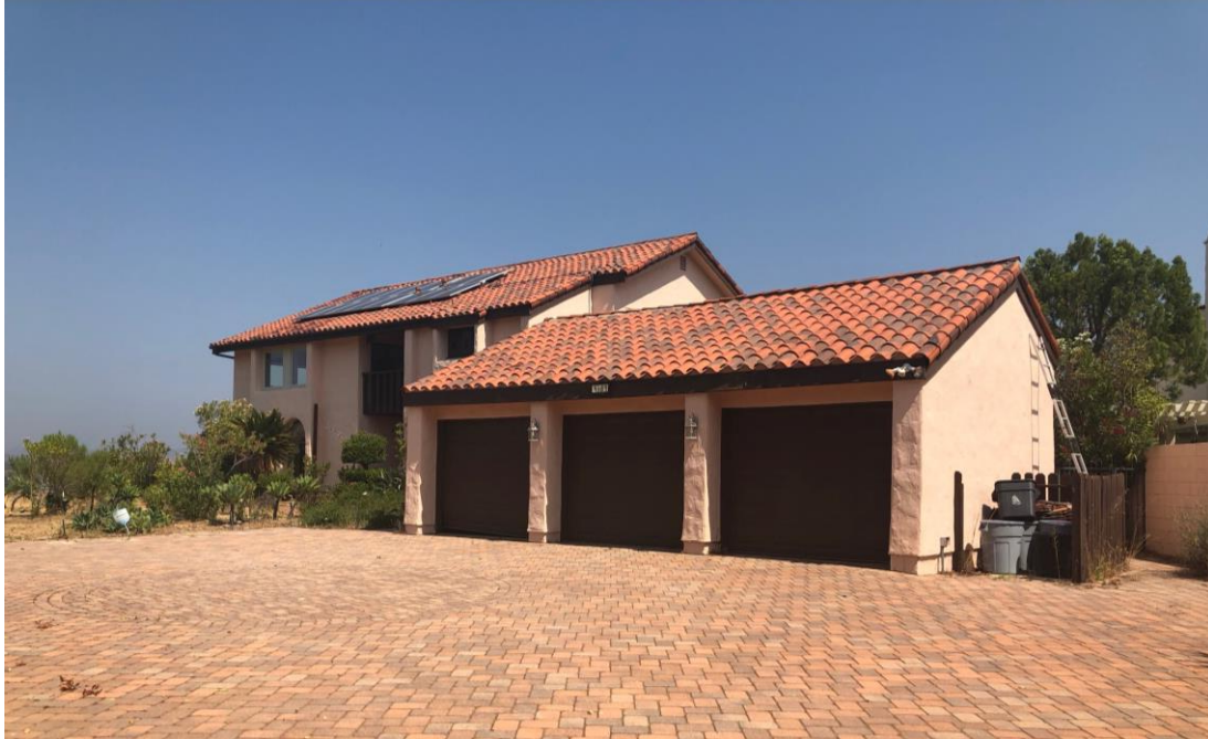
Standing on the driveway of the subject site looking at the existing two-story house to be demolished, facing northwest.
