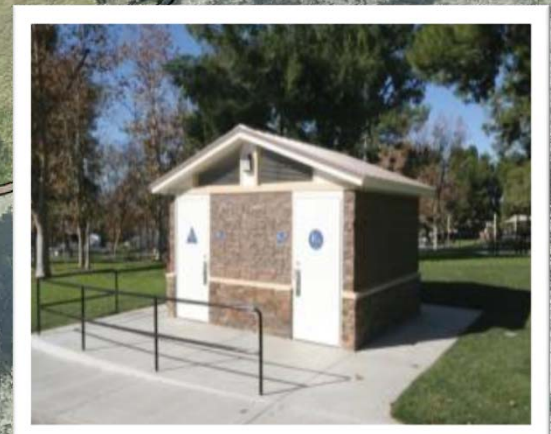
Permanent Restroom Building
