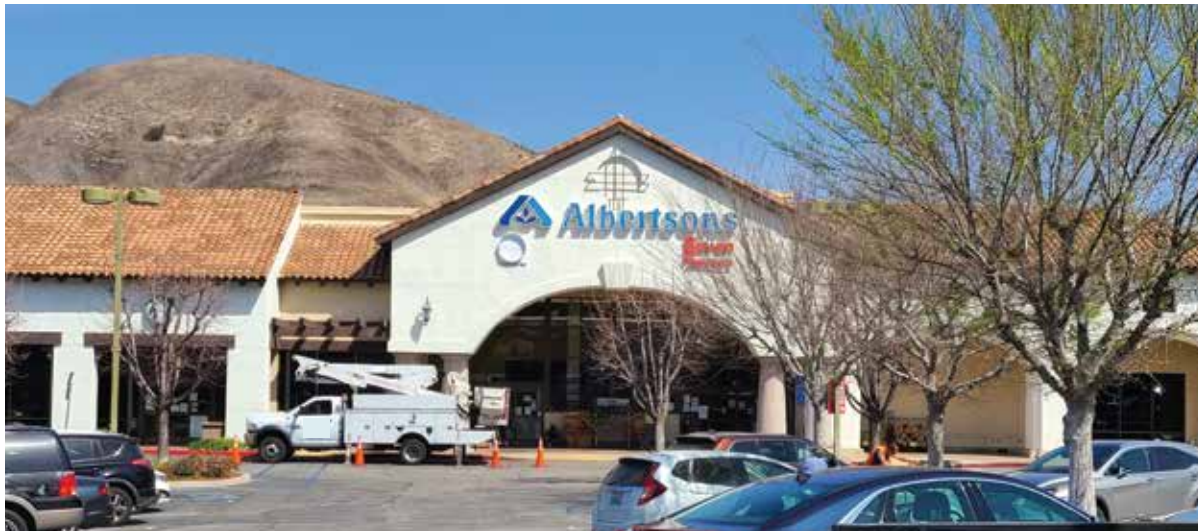
PRIMARY (PARKING LOT FACING SIGN)
