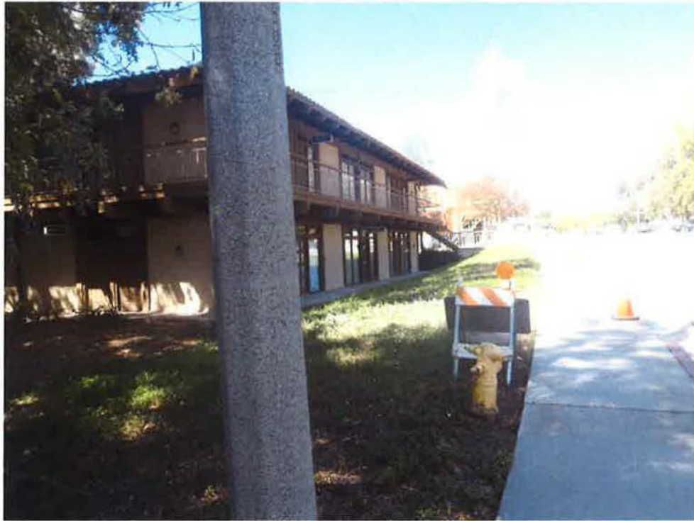
Photograph 1: overview to west from northeast corner 23480 Park Sorrento.
