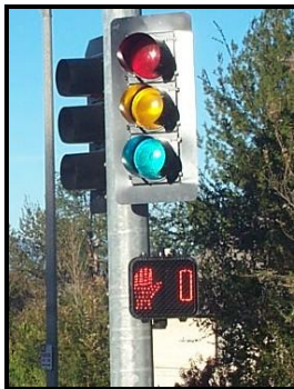
Pedestrian Countdown Signal at Paul Revere Drive
