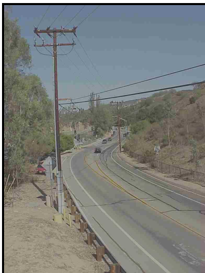
Calabasas High School Frontage on Mulholland Highway
