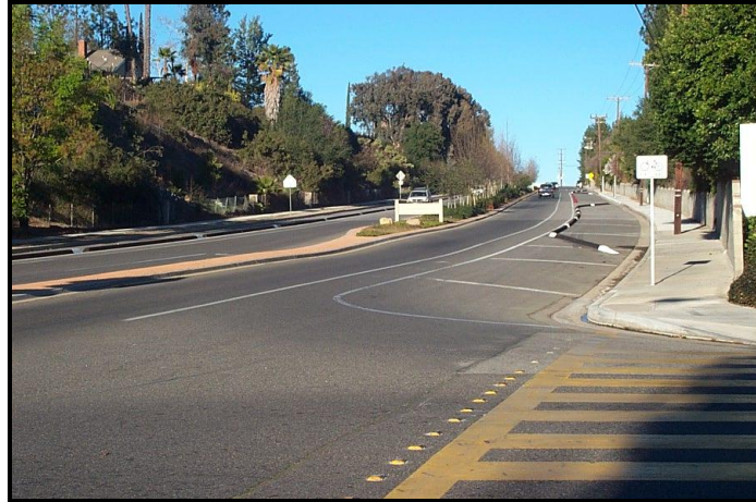
View of the Corridor Looking East from Eddingham Avenue
