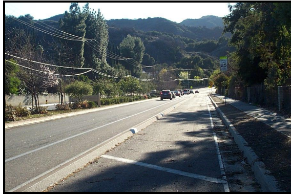
New Asphalt Berm near Daguerre Drive
