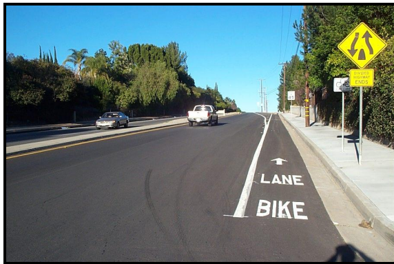
Existing Middle Segment of Zone 2
