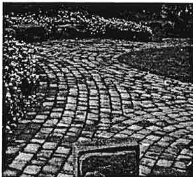
"Terra Craft" cobble stone pavers in San Francisco color used in cross walks.
