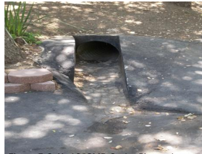
Figure 5.2.1b 18" CMP Outlet Pipe at Locust Dr.
