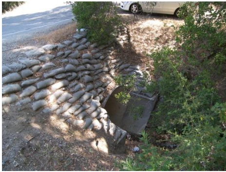
Figure 5.2.2a 72" RCP Culvert Inlet
