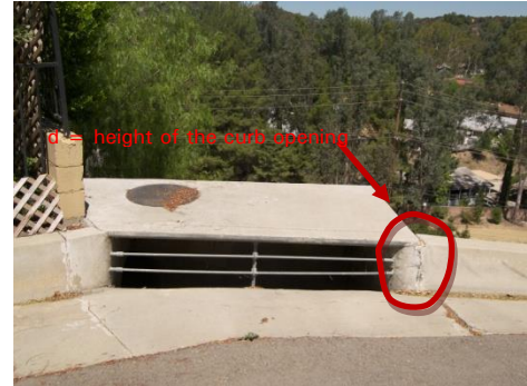
Figure 4.2.2.2a Curb-Opening inlet in Pansy Tr.
