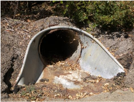
Figure 4.2.1.3a CMP Culvert Inlet in Daisy Trail.
