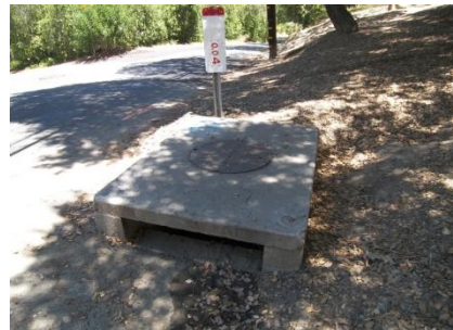
Figure 5.2.1d 24" CMP Catch Basin at Valley View Rd.
