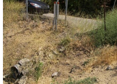
Figure 5.2.6b 18" CMP Outlet Adjacent to Summit Dr.
