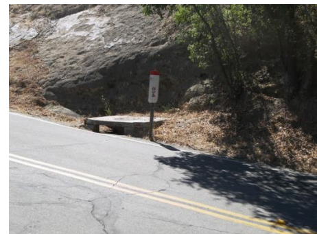
Figure 5.2.2b Inlet on Canyon Dr.
