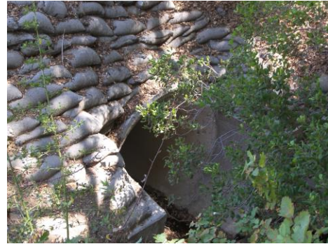
Figure 4.2.1.3b RCP Culvert Inlet in Canyon Drive.
