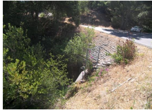
Figure 5.2.2b 72" RCP Culvert Outlet
