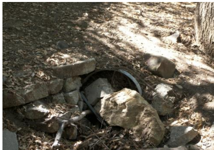
Figure 5.2.1c 24" CMP Outlet at Valley View Rd.
