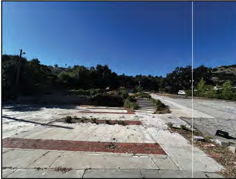
Photo 1A - Representative photograph of the northernmost portion of the Survey Area showing past development footprint and hardscaping.
