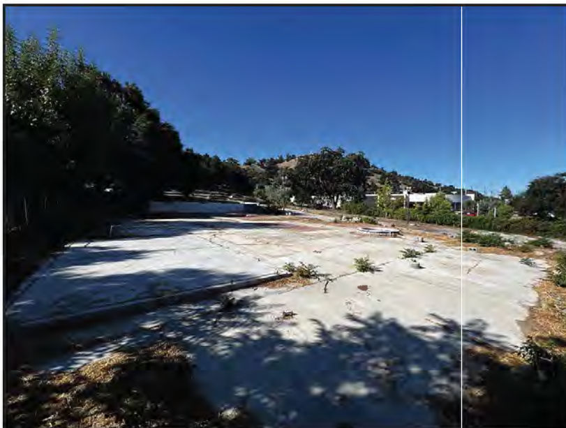
Photo 1C - Photograph of hardscaped area in the northern portion of the Survey Area.
