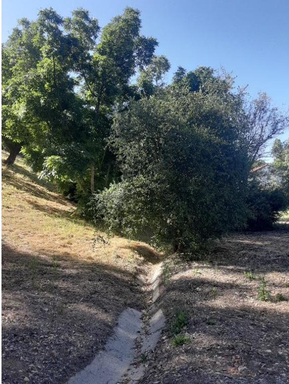
Lower end of brow ditch
