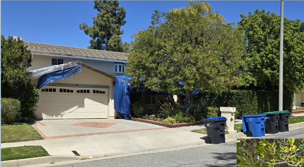
Front of house as viewed from street
