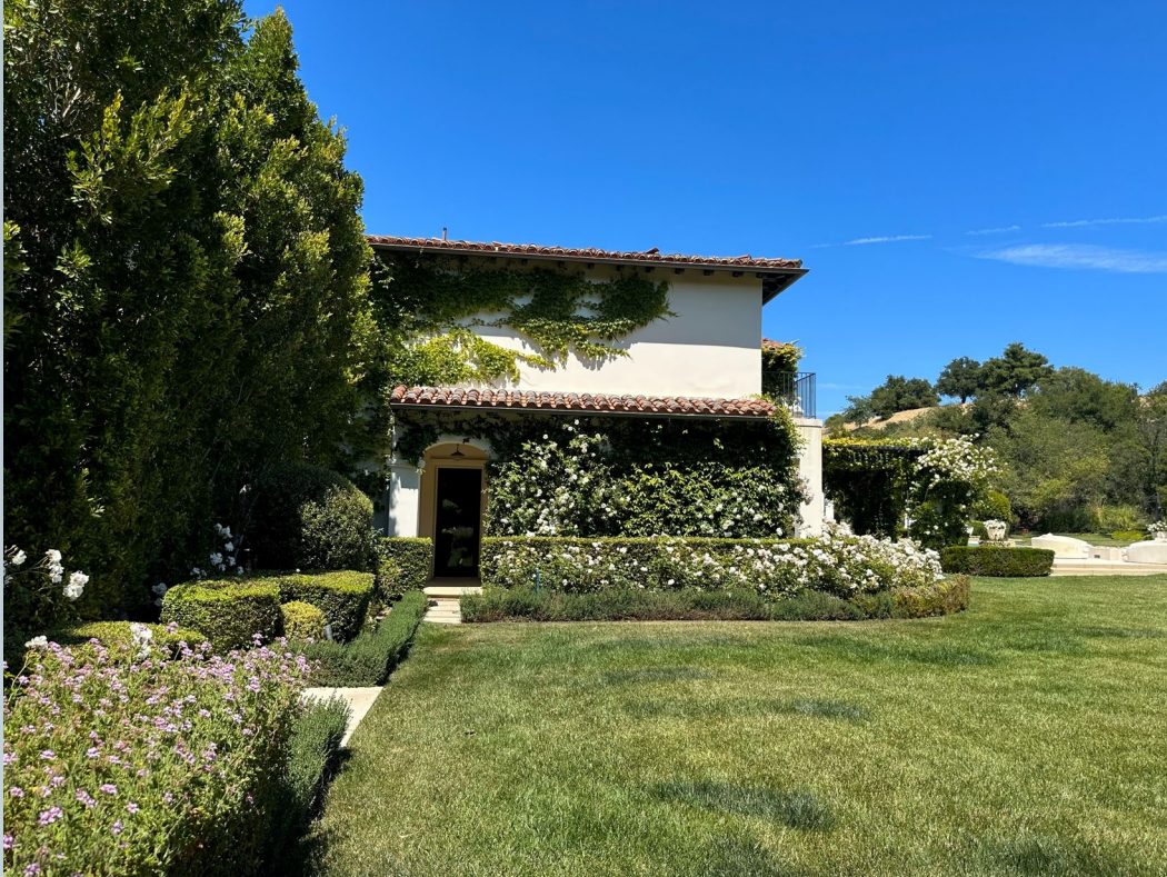
West side of house (location of proposed addition)
