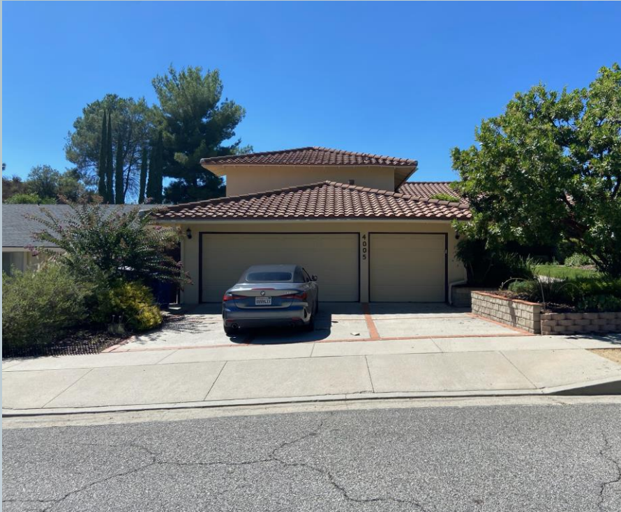
Front of house as viewed from street
