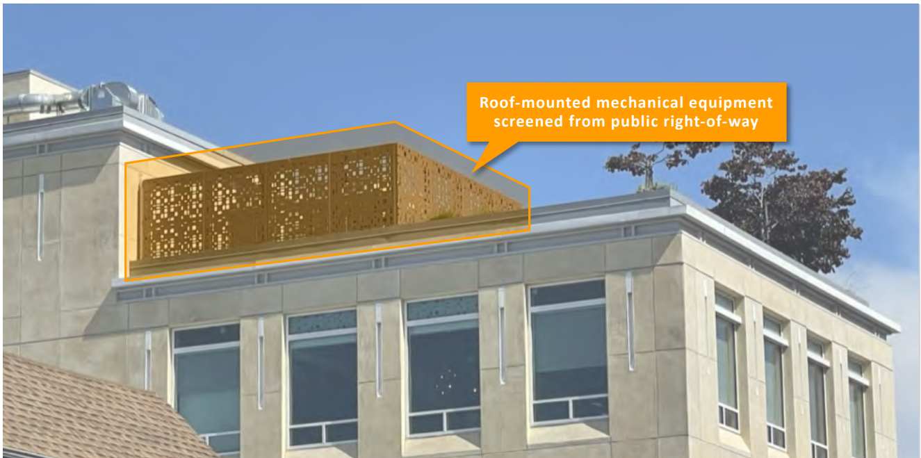
Figure 56: Roof mounted mechanical equipment shall be screened so it is not visible from the adjacent public right of way. (Section 6.3.C)
