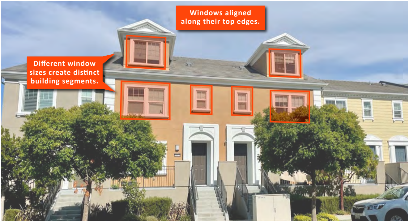
Figure 27: Differing window sizes and alignment of windows along their top edges create distinct building segments. (Section 4.1.6.B)
