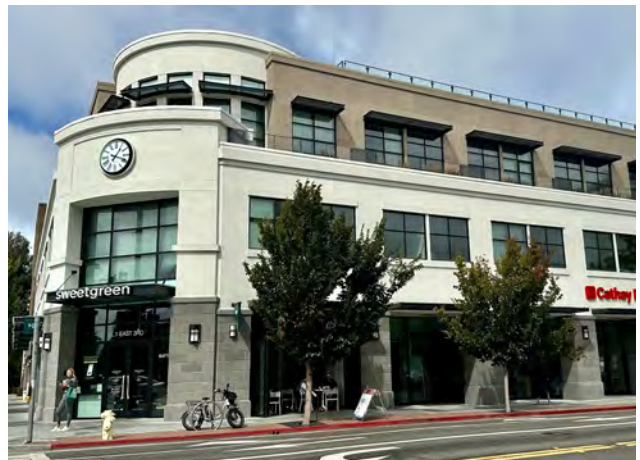
Figure 70: Minimum four (4)-foot stepback above the second story (Section 7.5.1.A)
