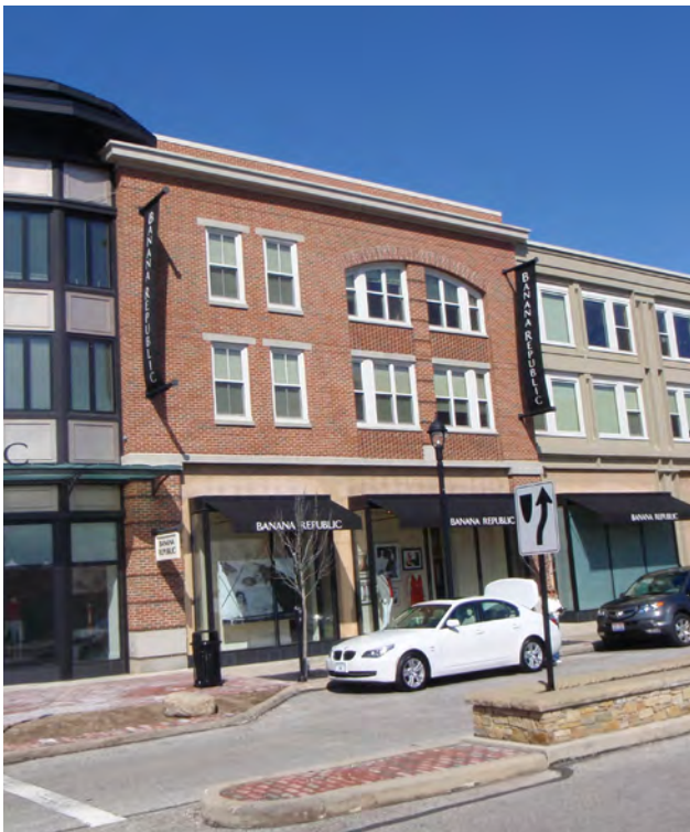
Figure 44: Individual entry for tenants in retail/commercial or other non-residential entry design (Section 4.6.5.C)
