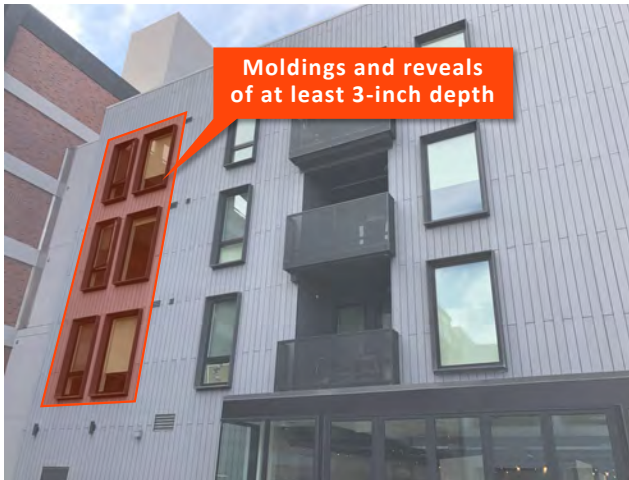
Figure 40: Window recesses and edges, including molding and reveals of at least three (3)-inch depth (Section 4.6.2)
