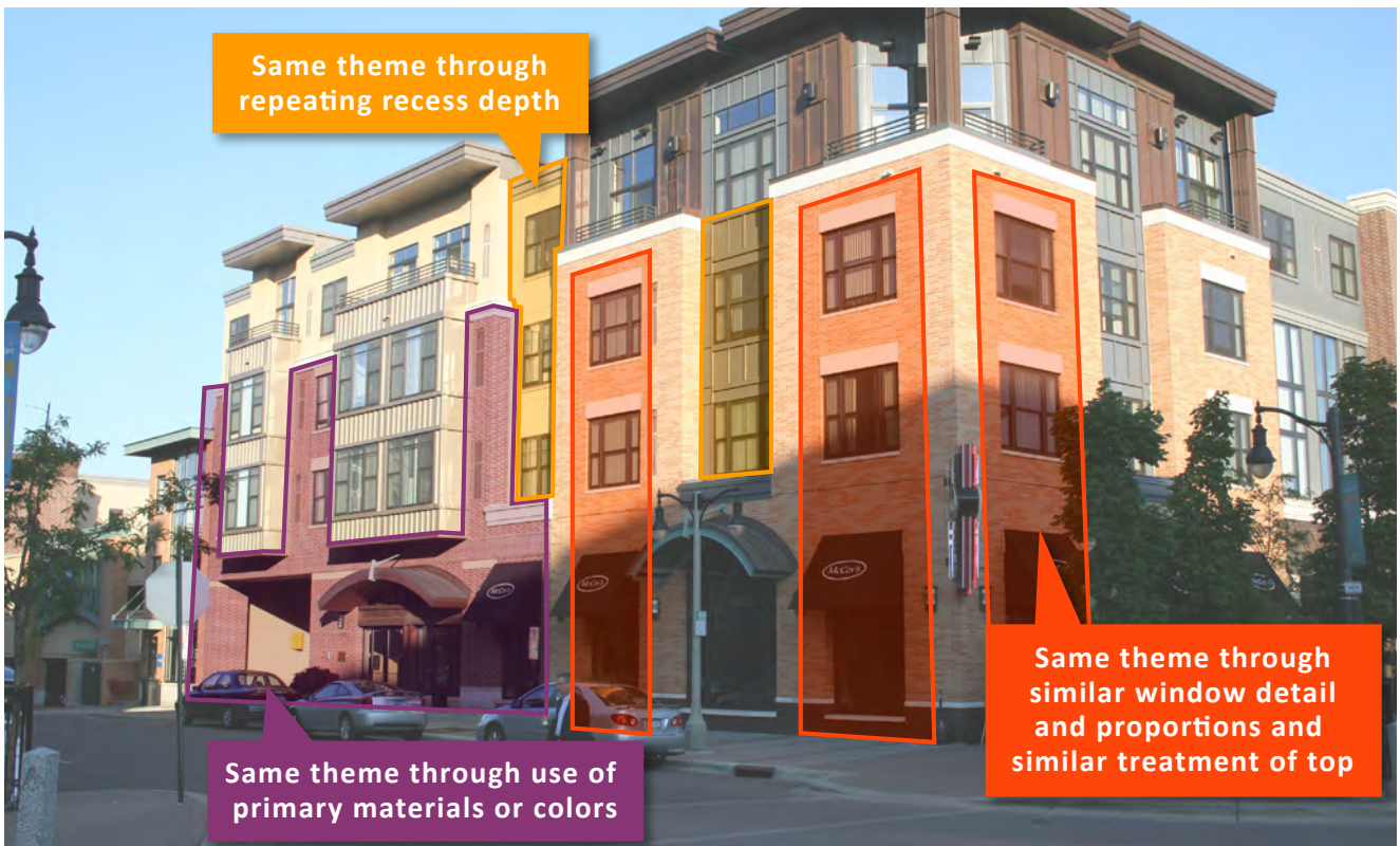
Figure 34: Mixed use buildings demonstrate consistent design on all elevations through the use of primary materials or colors, similar window detail and proportions, and similar treatment of top. (Section 4.3.1)
