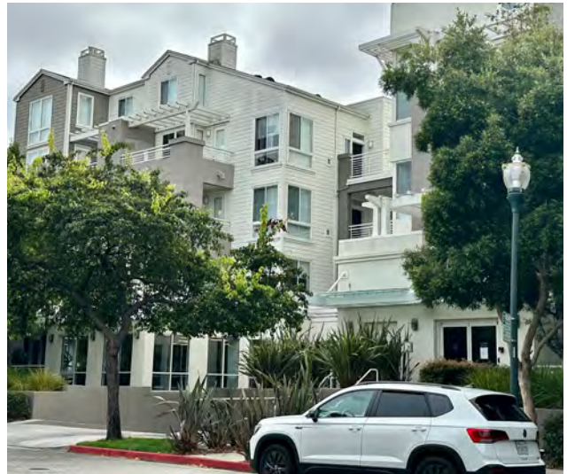
Figure 64: A minimum four (4)-foot stepback shall be provided above the second story. (Section 7.2.3)
