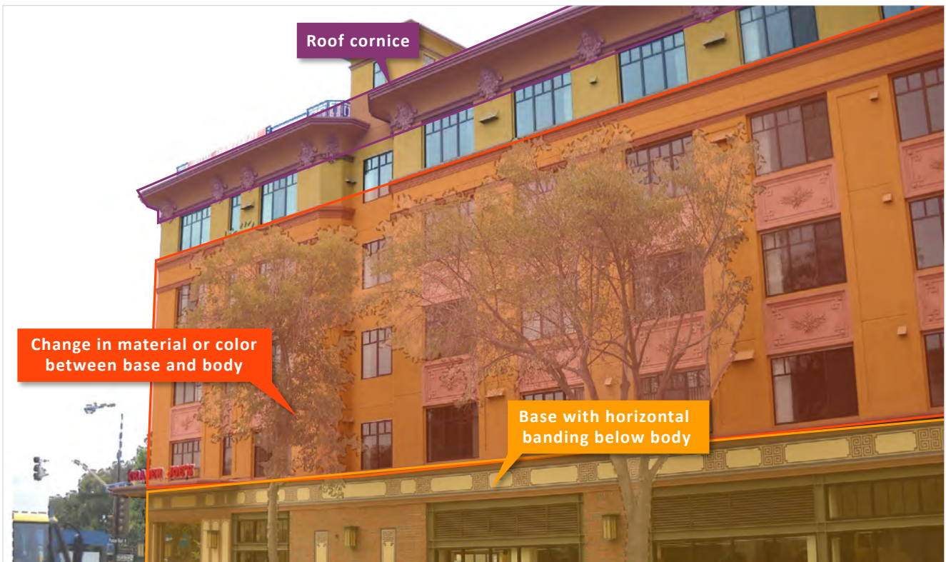
Figure 25: Vertical wall plane breaks can be accomplished by incorporating a roof cornice or change in material or color between the base and body. (Section 4.1.6.B)
