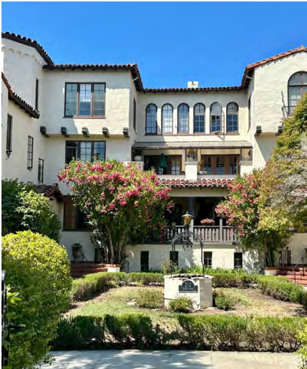
Figure 58: Building facing of light-colored stucco shall be used to achieve a Spanish Colonial Revival architectural style. (Section 7.1.2)
