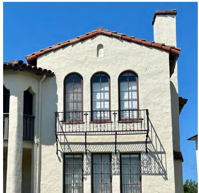
Figure 39: Grouped windows with a minimum of three inches of building façade surface between them (Section 4.6.1)
