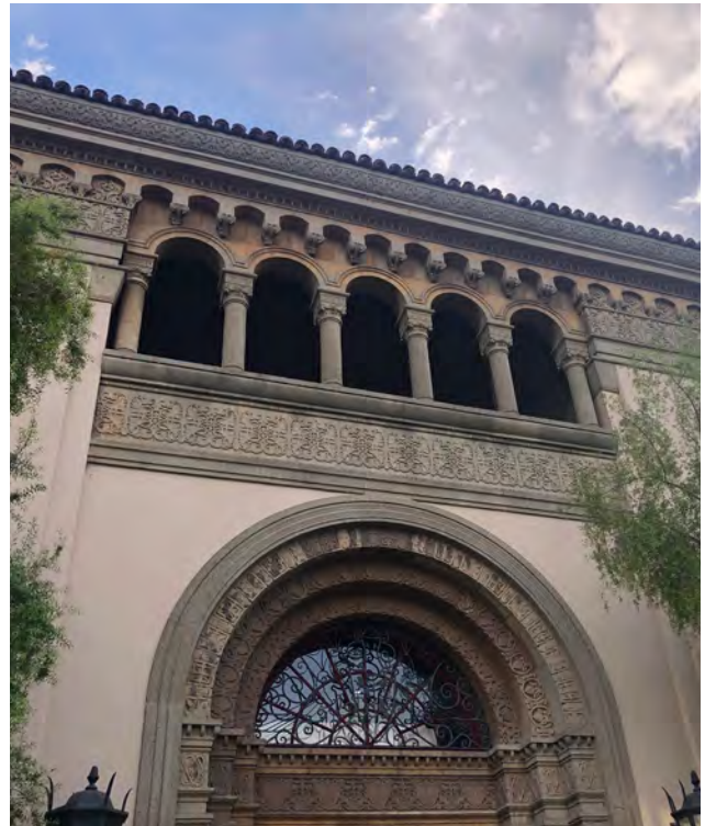
Figure 59: Tile and stone are acceptable materials to use to achieve a Spanish Colonial Revival architectural style. (Section 7.1.2)
