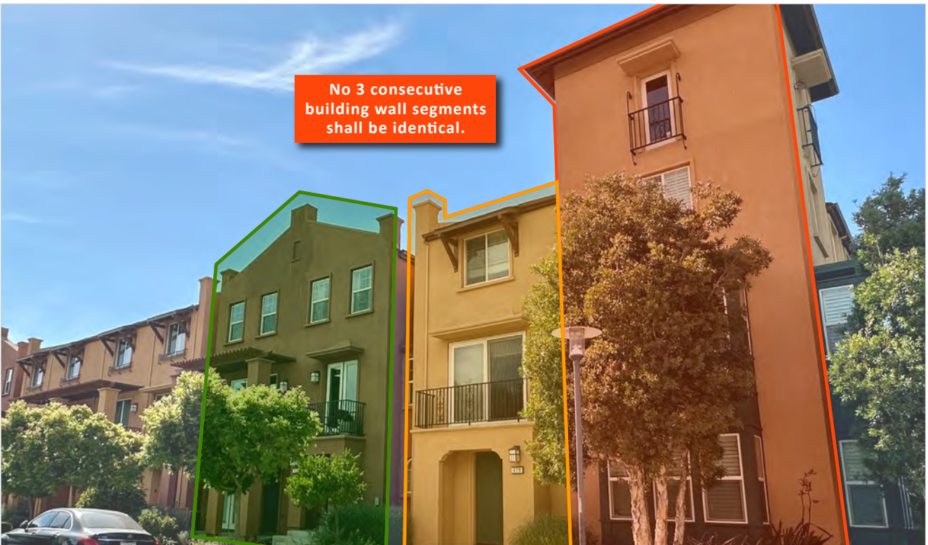
Figure 28: To prevent repetitive wall designs, no three (3) consecutive building wall segments shall be identical.
