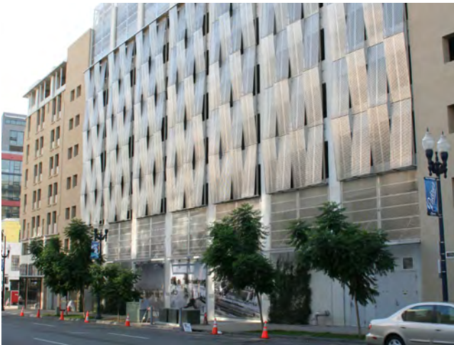
Figure 16: Decorative screening elements screen the parking structure from the public right-of-way. (Section 3.2.4.C.3)
