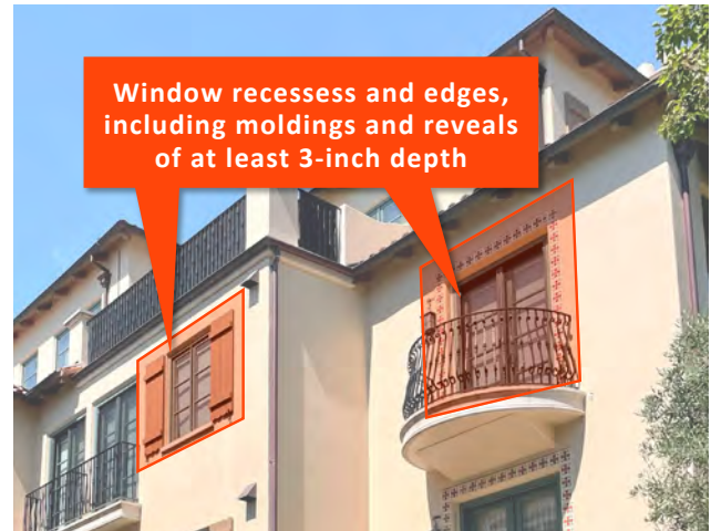
Figure 41: Window recesses and edges, including moldings and reveals of at least three (3)-inch depth (Section 4.6.2)
