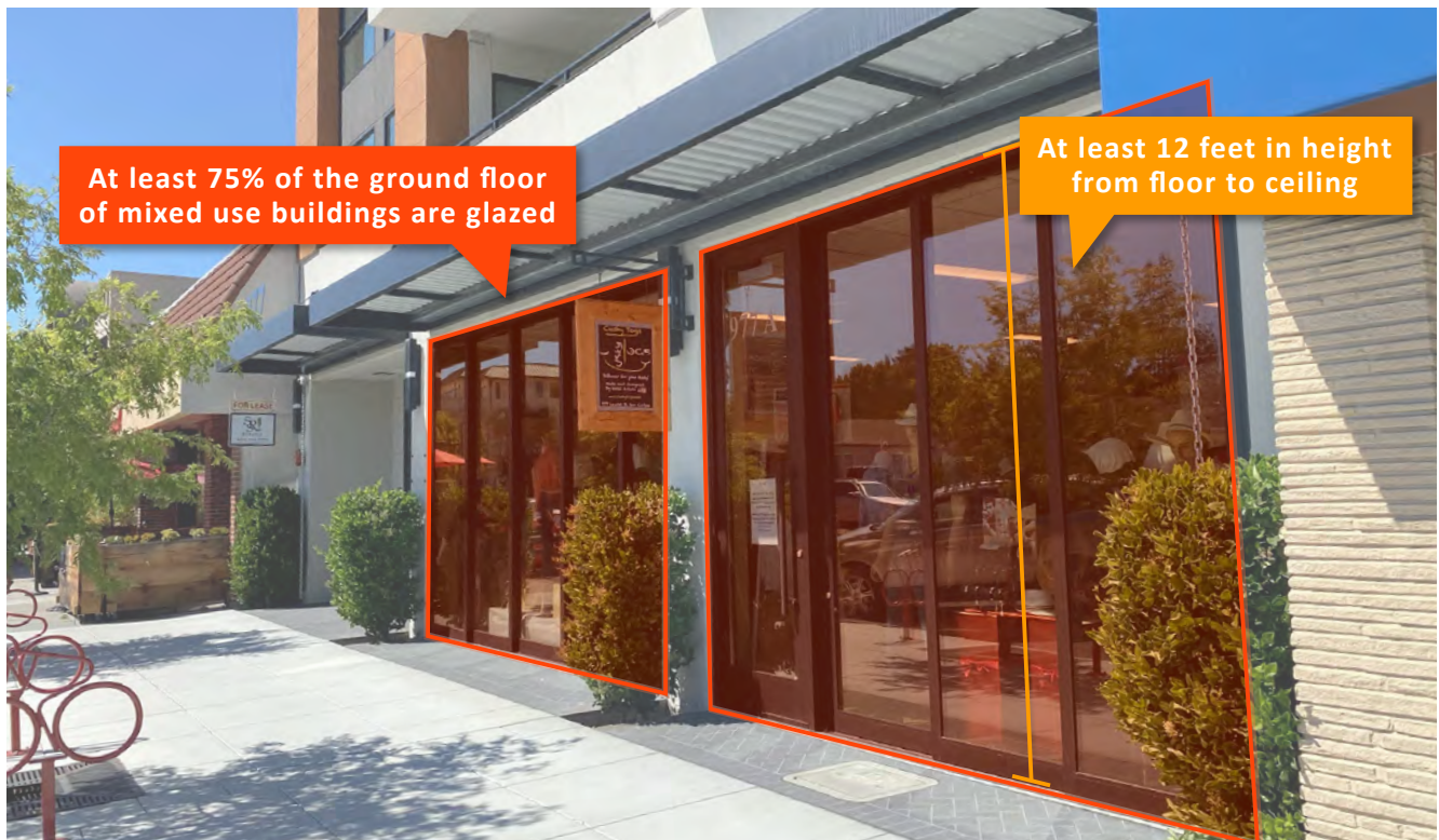
Figure 33: Ground floor commercial uses shall be at least 12 feet in height. (Section 4.2.1.B)
