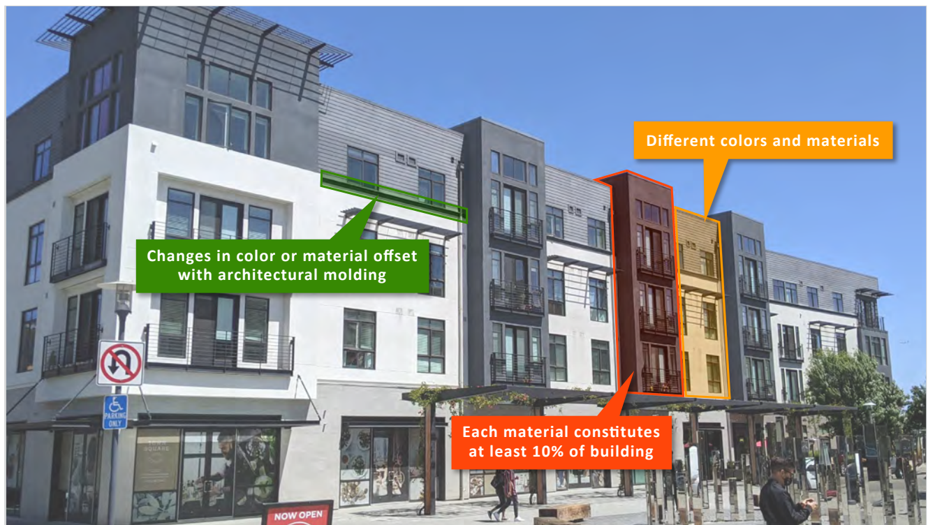
Figure 20: A mid-rise building with different colors and materials on the building façade to avoid a monochromatic color scheme and use of materials. (Section 4.1.3)
