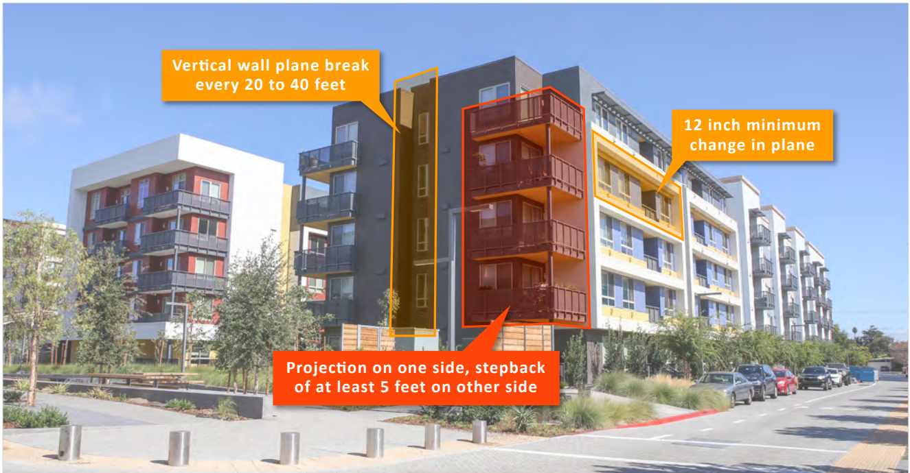
Figure 24: Wall plane treatments shall be incorporated into the design of mid-rise buildings. (Section 4.1.6.B)
