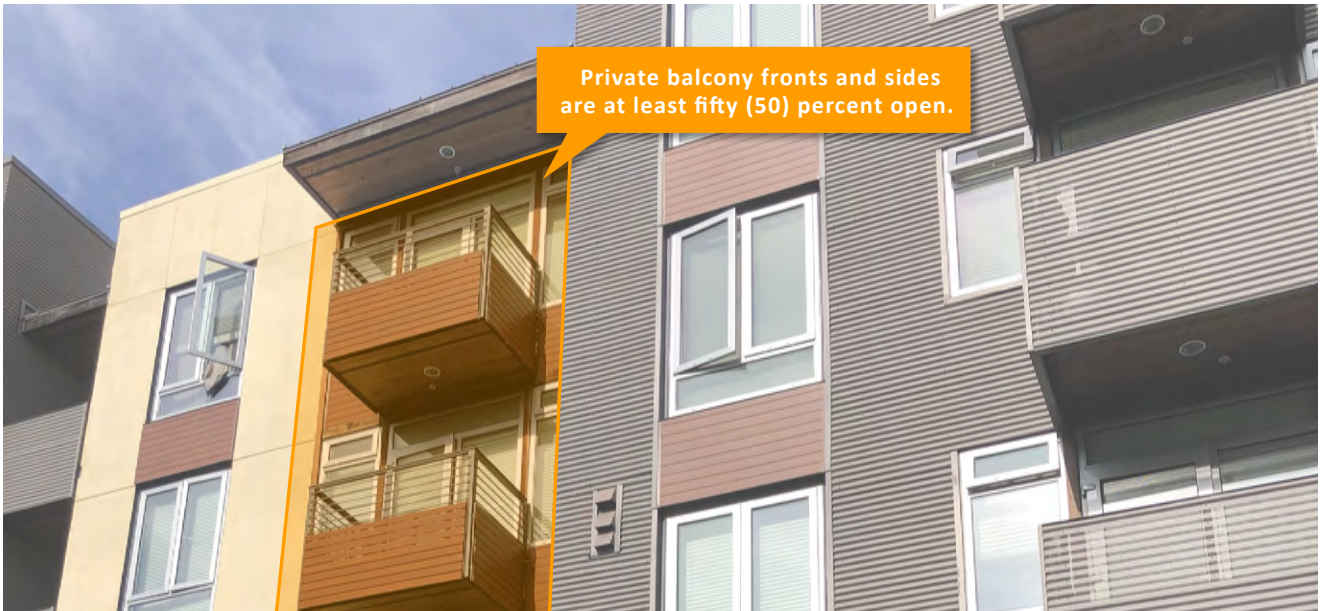
Figure 50: The fronts and sides of balconies shall consist of obscured glass, slats, or partially transparent grating or railing that is at least fifty (50) percent open. (Section 5.1.1.B)
