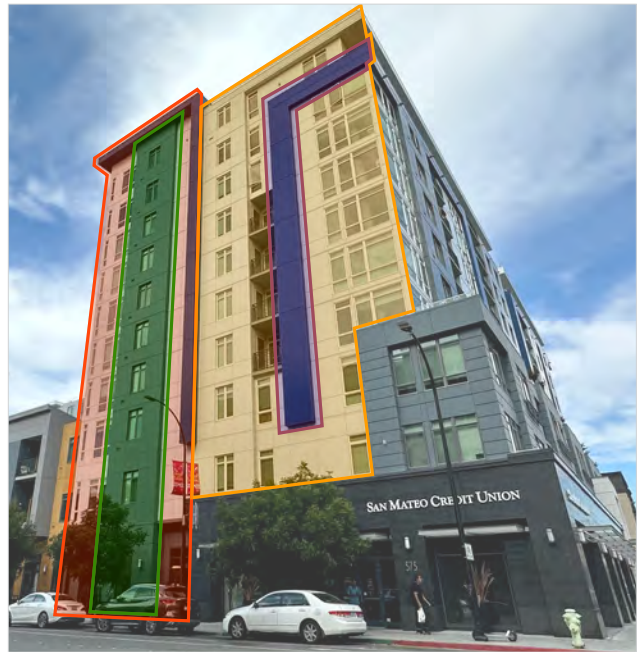
Figure 32: To prevent repetitive wall designs, no two (2) contiguous building wall segments shall be identical.
