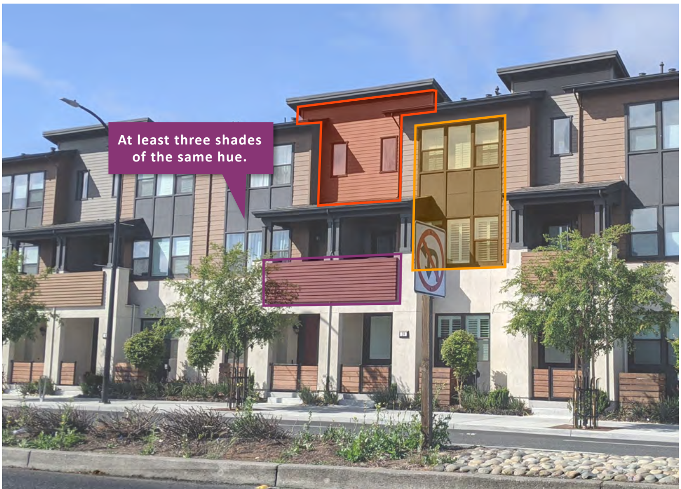
Figure 47: Colors of the same hue shall be differentiated by at least three shades. (Section 4.7.1.A)
