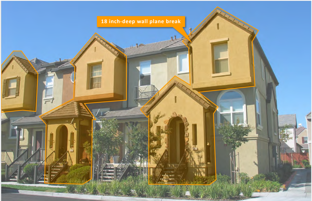
Figure 22: Low-rise buildings shall have a minimum eighteen (18) inch-deep wall plane break for every fifteen (15) to thirty (30) feet of horizontal wall length. (Section 4.1.5)
