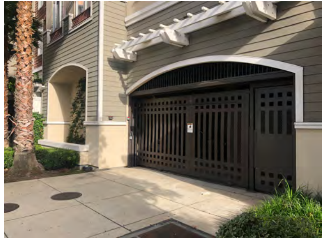
Figure 46: Minimum six (6) inch recess (Section 4.6.5.D)
