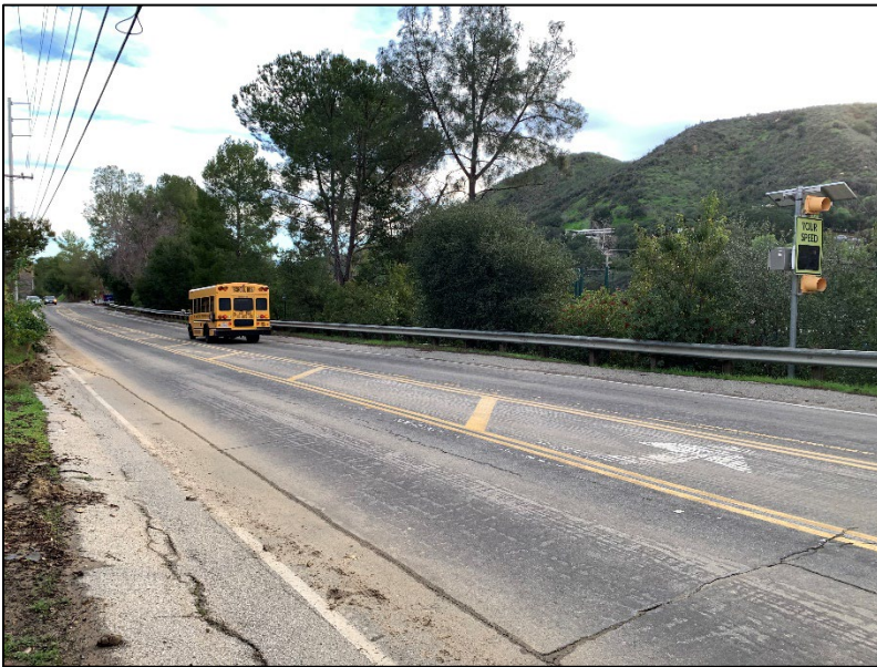
a. Caisson retaining wall site at Viewpoint School
