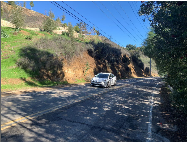
c. Slope to be stabilized with steel netting, north of Parksouth Street
