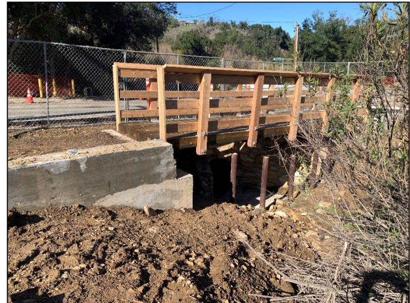
d. Culvert improvement site, east (upstream) of Mulholland Highway
