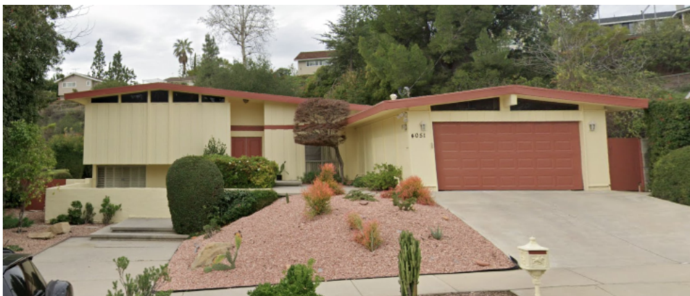
EXISTING FRONT VIEW
