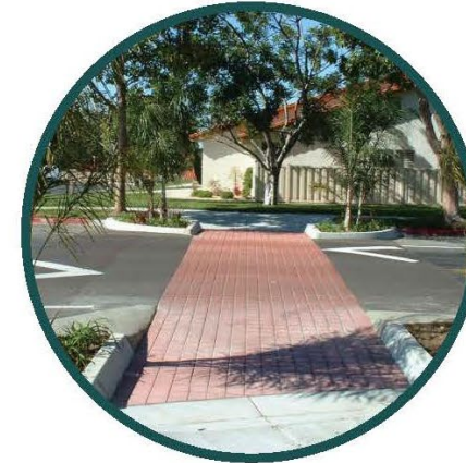
Raised Crossings & Intersections
