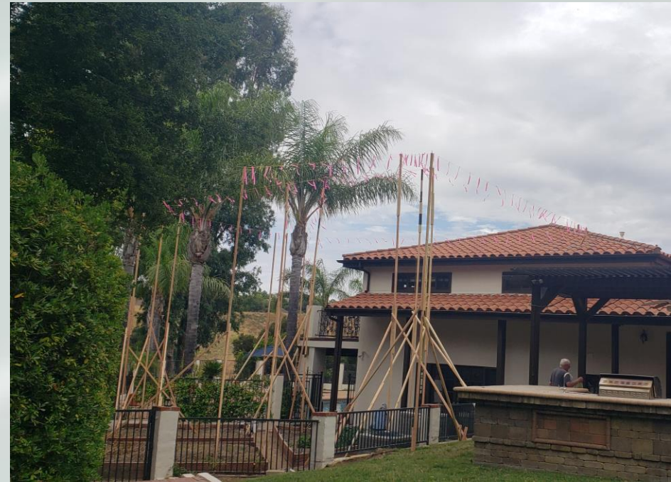
View from rear yard of subject site
