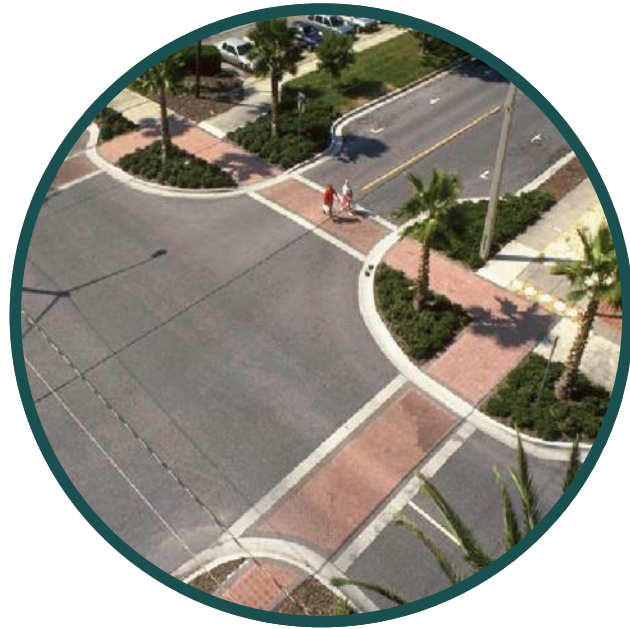
Corner Extensions (pending fire dept. approval)
