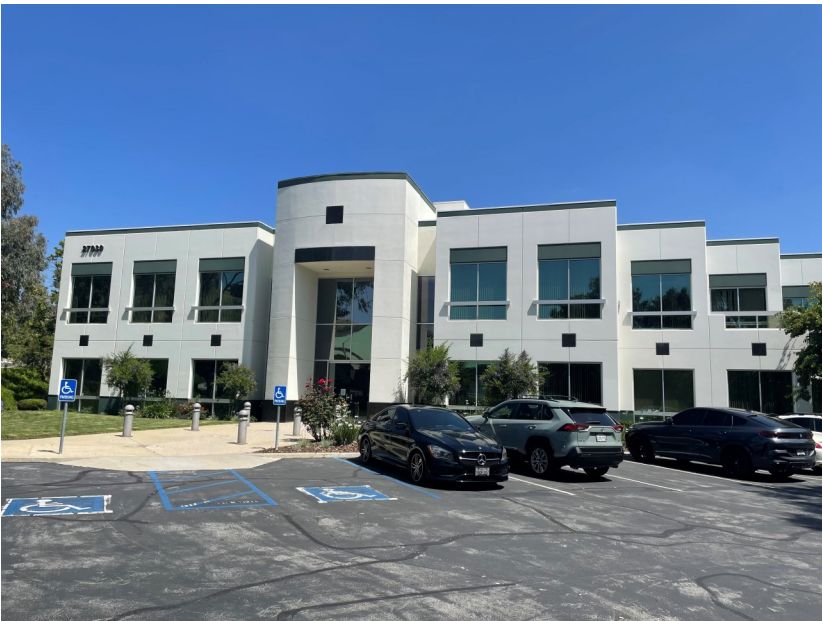
COMMERCIAL BUILDING ACROSS THE STREET FROM THE COMMUNITY CENTER
