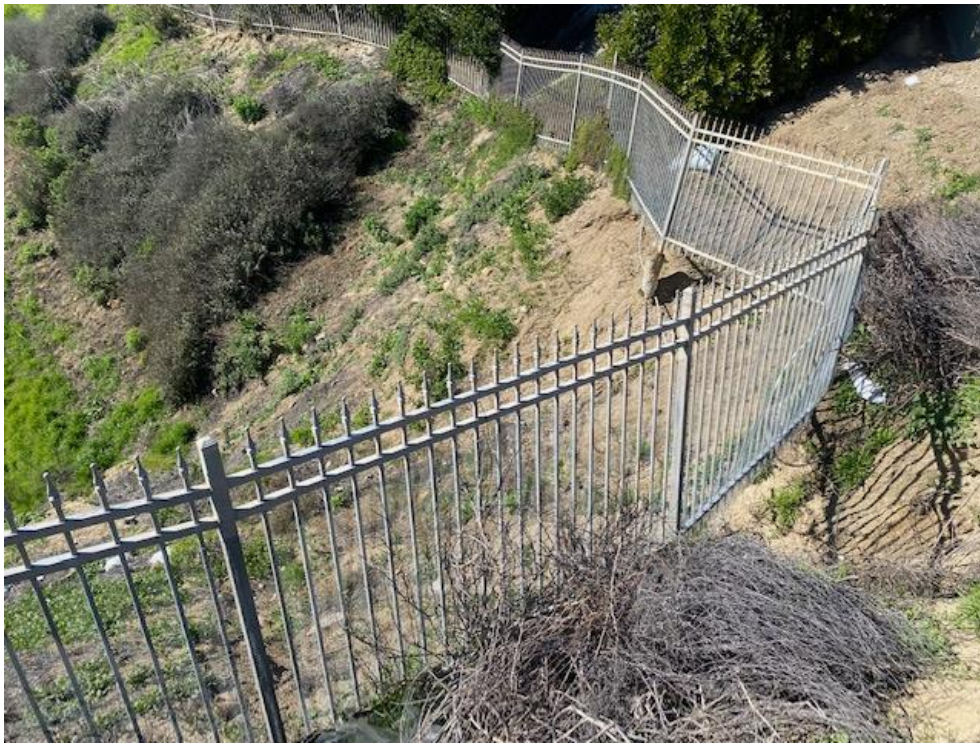
Photos 1-4: Taken prior to recent rain, depicting visible fence footings
