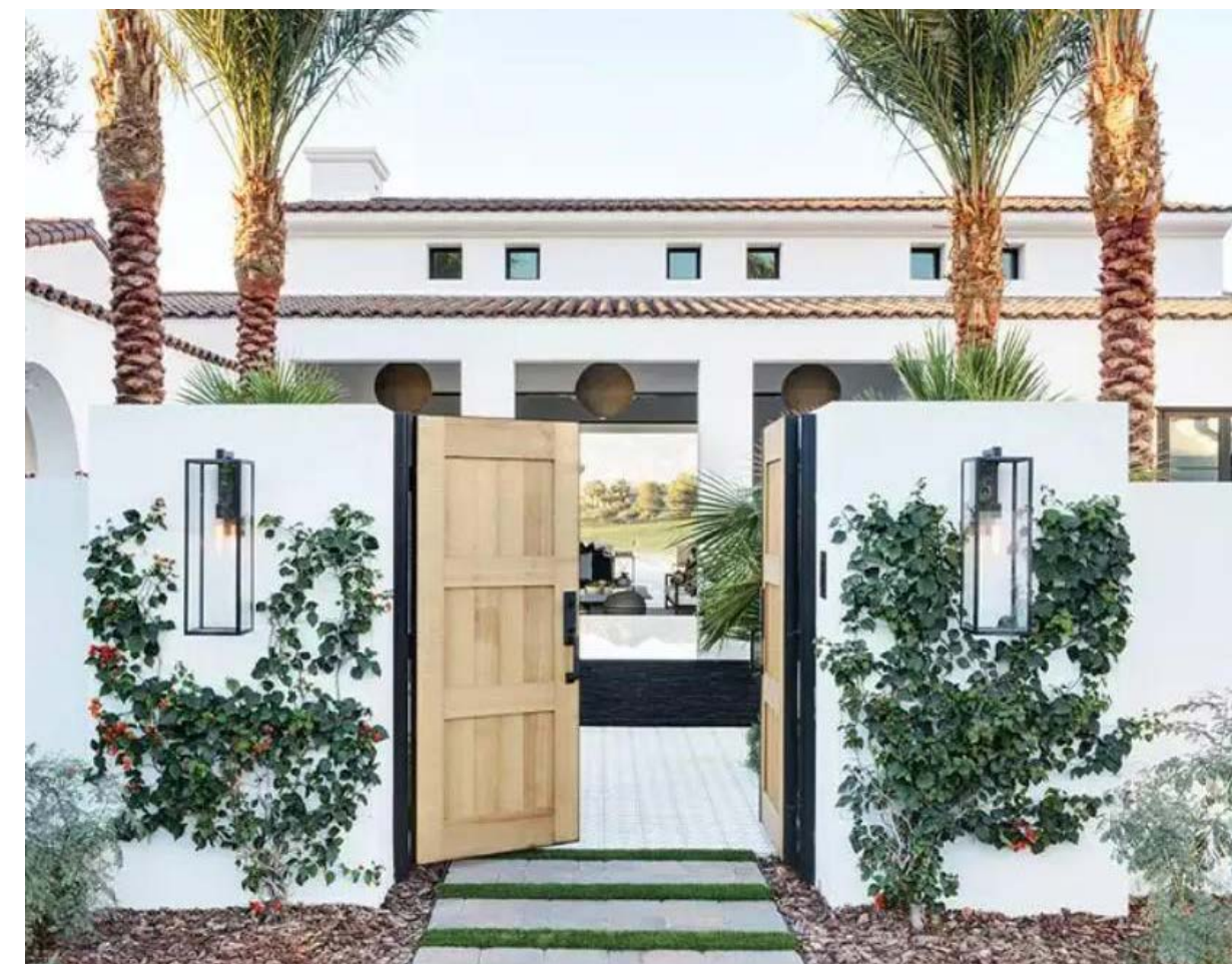
GARAGE DOOR & GATE SOLID WOOD STAINED & SEALED WEATHERED WOOD FINISH
