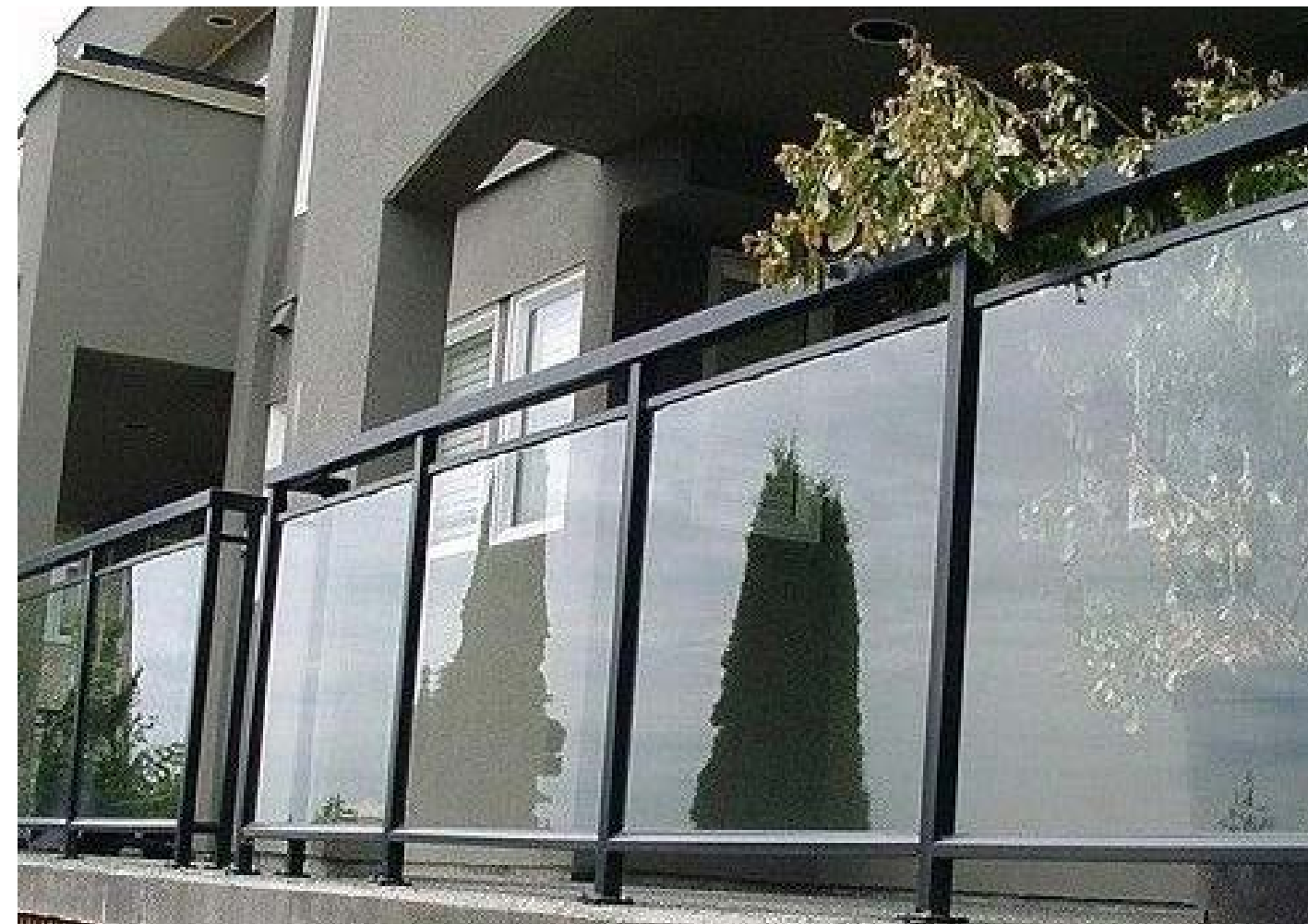
RAILING BLACK METAL FRAME WITH TEMPERED GLASS PANELS COLOR: BLACK
