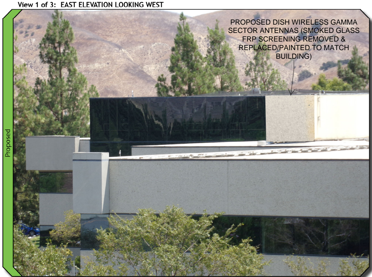
View 1 of 3: EAST ELEVATION LOOKING WEST
