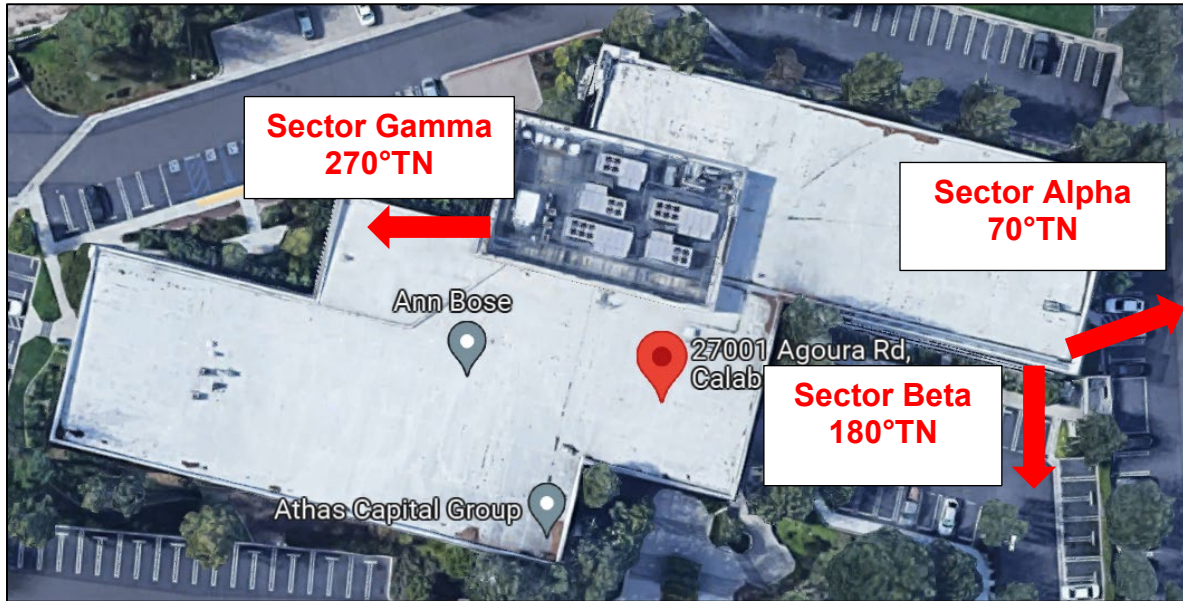
Figure 1: Overview of existing building and approximate sectors (Source: Google Maps Capture 2022; annotations by Dr. Kramer).
