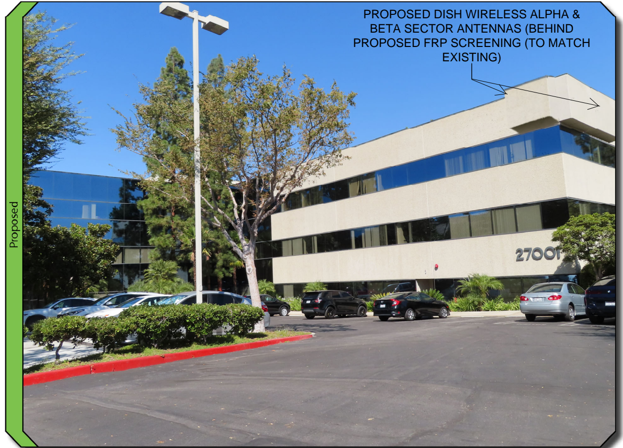
View 2 of 3: SOUTH ELEVATION LOOKING NORTH
