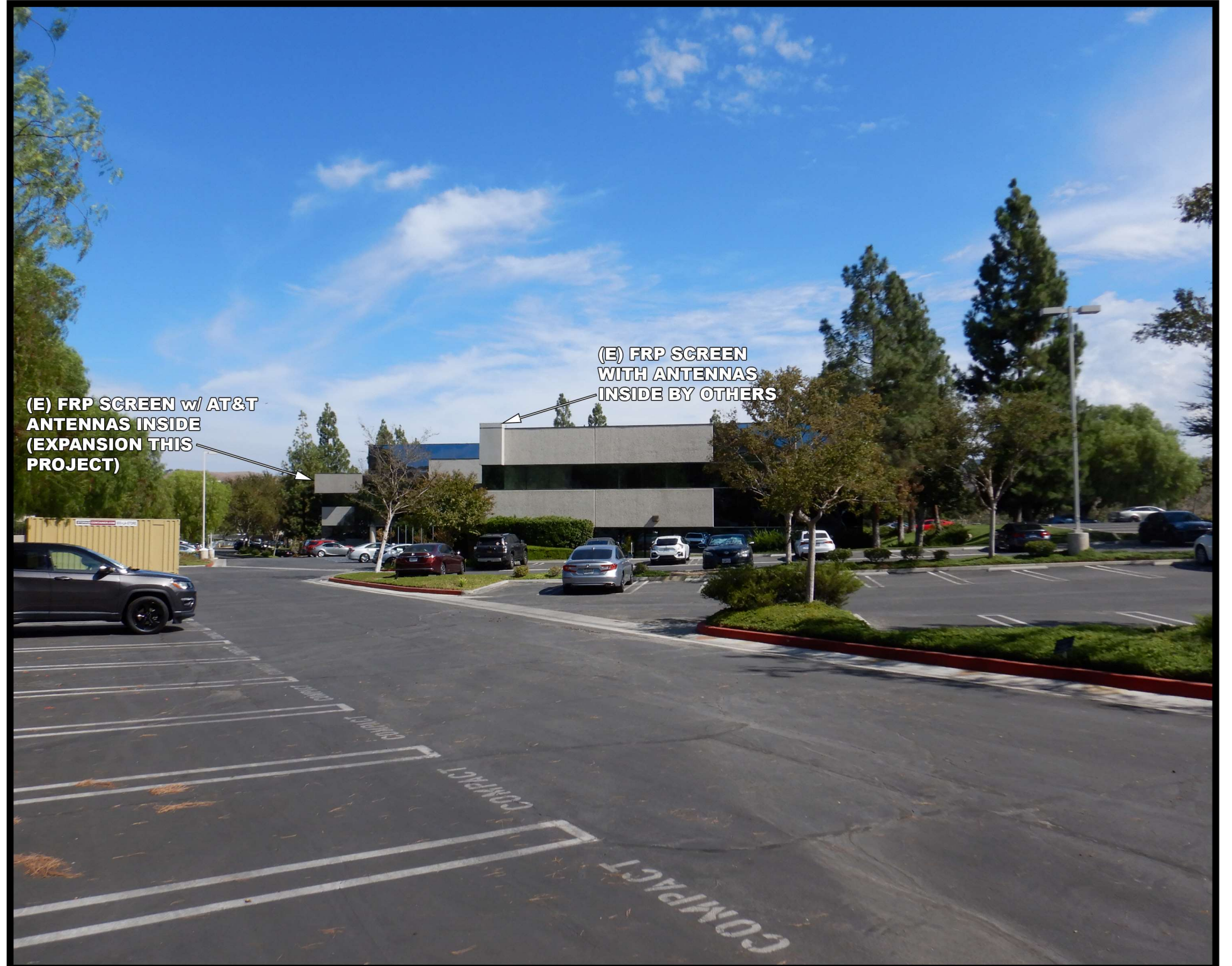
VIEW FROM WEST OF (E) BUILDING
