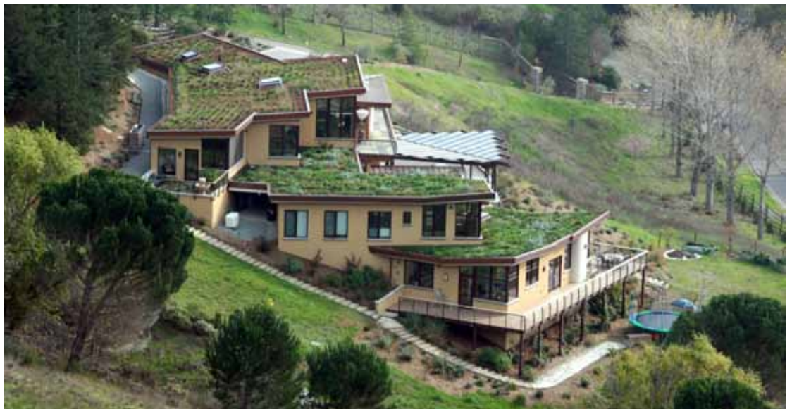
Mill Valley home with green roof
