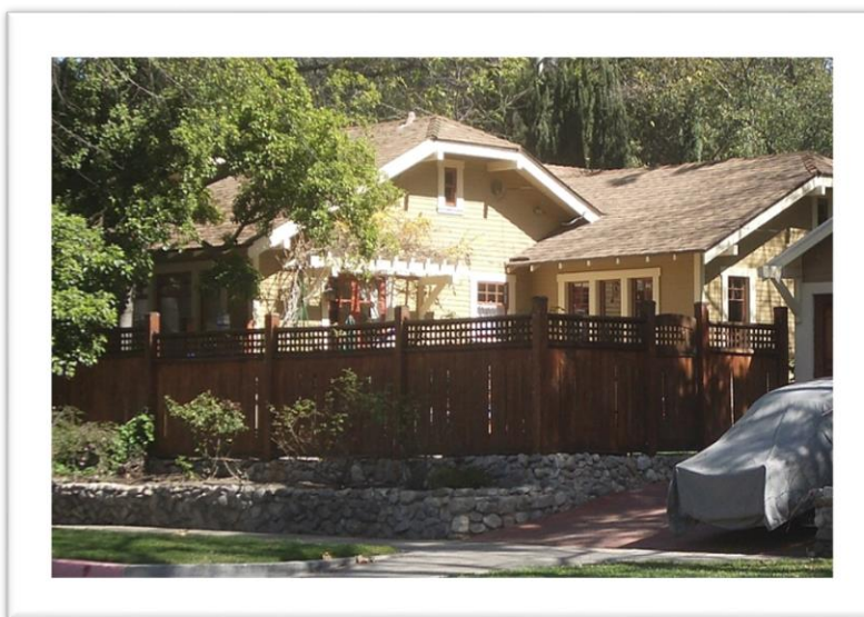
Figure 29 - Claremont house remodel
