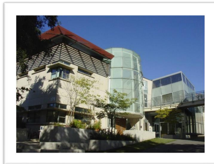
Figure 21 – LEED-certified building: Pomona College
