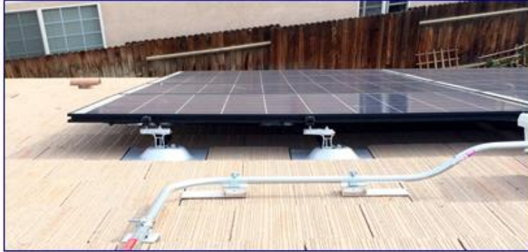
“After” – Supported per installation instructions
