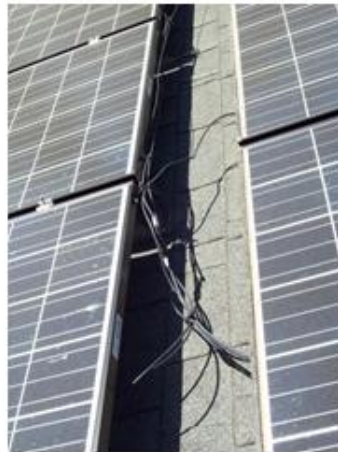
POORLY ROUTED AND UNSECURED – “LAYING ON ROOF SURFACE AND VENT”
