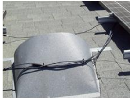
POORLY ROUTED AND UNSECURED – “LAYING ON ROOF SURFACE AND VENT”
