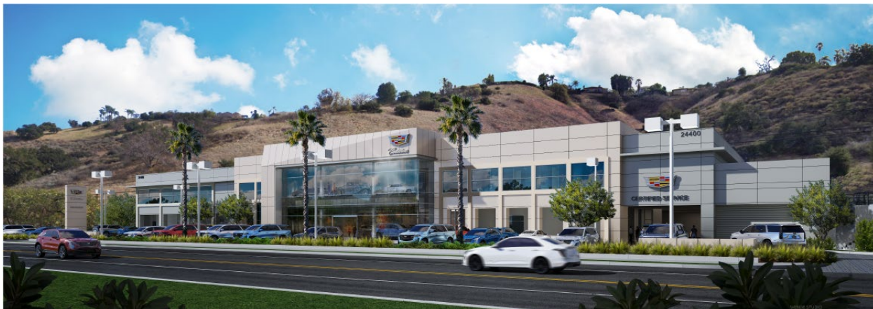
(Image 2: Daytime Rendering depicting the updated design changes incorporating the Panel's recommendations).
