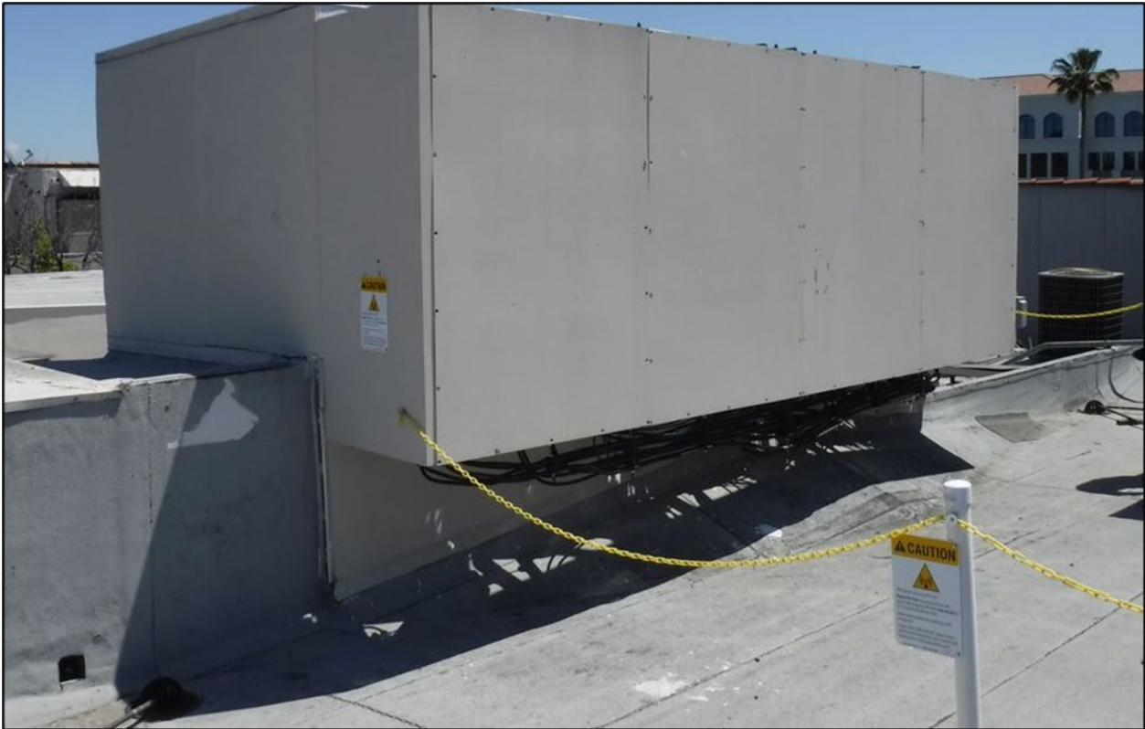
Figure 5: Existing barriers on rooftop (Source: Applicant Photos).
