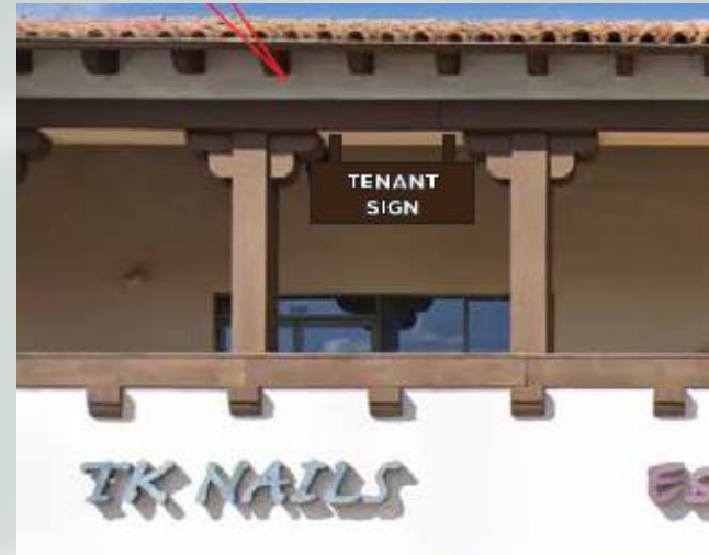
Revised proposal. 11 SF hanging sign mounted to existing wood beam, reviewed by ARP on November 19, 2021.
