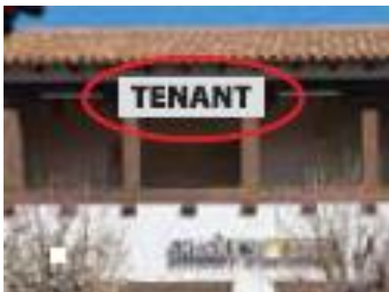
Figure 1: Initial proposal. 20 SF sign mounted to existing support posts in front of corbels, reviewed by ARP on July 23, 2021.
