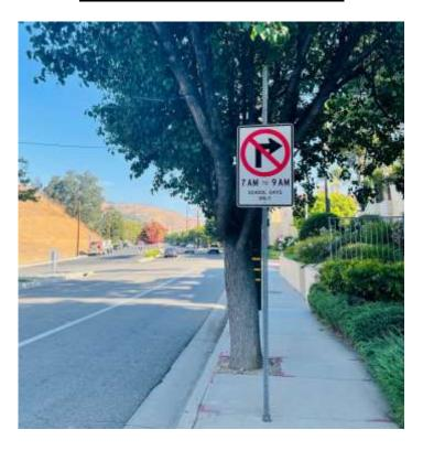
Description: Turning movement restrictions utilize signs to prevent undesired turning movements without the use of physical devise. These signs could be installed to reduce vehicle movements by time of day or all day to address specific issues for cut-through traffic concerns. May require City Council approval of resolution for posting of restrictions.
