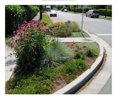
Description: A raised addition of sidewalk that extends the curb to effectively narrow the street at an intersection in order to reduce width of the traveled-way. Curb extensions can provide identity to a neighborhood by creating a gateway. They improve pedestrian comfort and safety by providing a better line of sight between the motorist and the pedestrian. The exact configuration of the treatment will depend upon the location and can be combined with a median.
