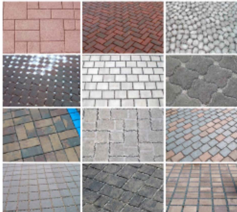
Figure 4-2 Various types of paving units used in PICP
