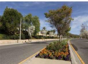
Description: A raised barrier which can narrow the driving lanes, eliminate turning movements, and eliminate straight-through traffic depending on the specific design. A median can take many forms to address the specific solution.
