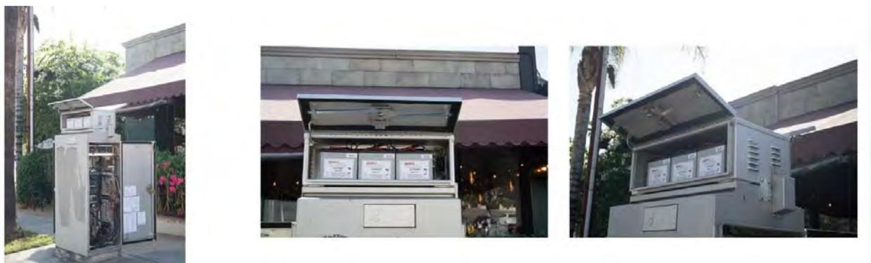
The internal mounted battery solutions will be placed on a tray within the cabinet so there will be nothing visible externally to compromise how the cabinets currently look.
