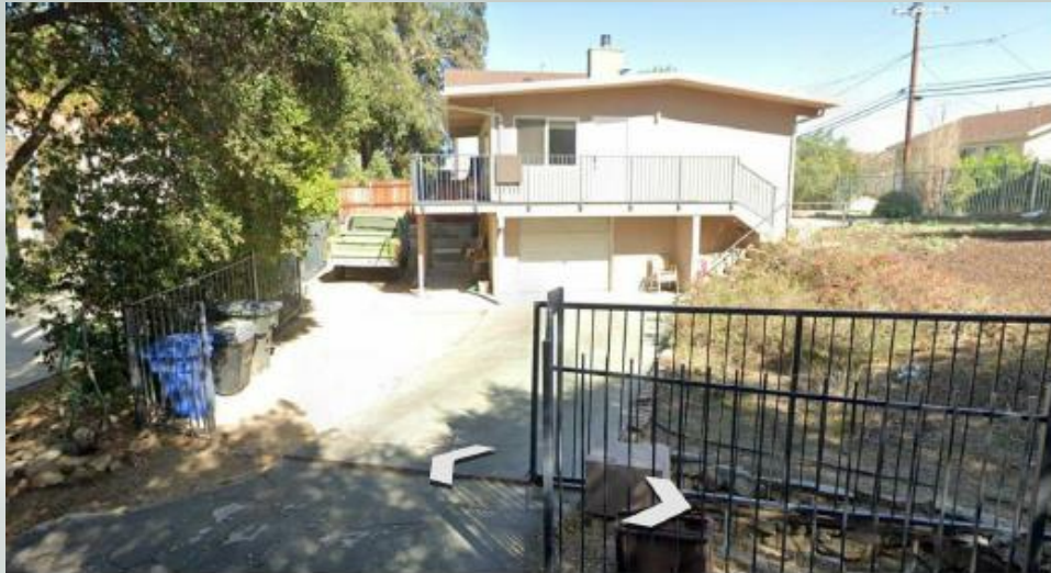
EXISTING VIEW FROM LOCUST
