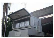
The internal mounted battery solutions will be placed on a tray within the cabinet so there will be nothing visible externally to compromise how the cabinets currently look.
